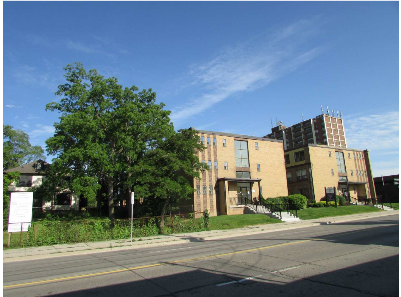
Photo 4 – Lands to the South, legal non-conforming apartment building.
