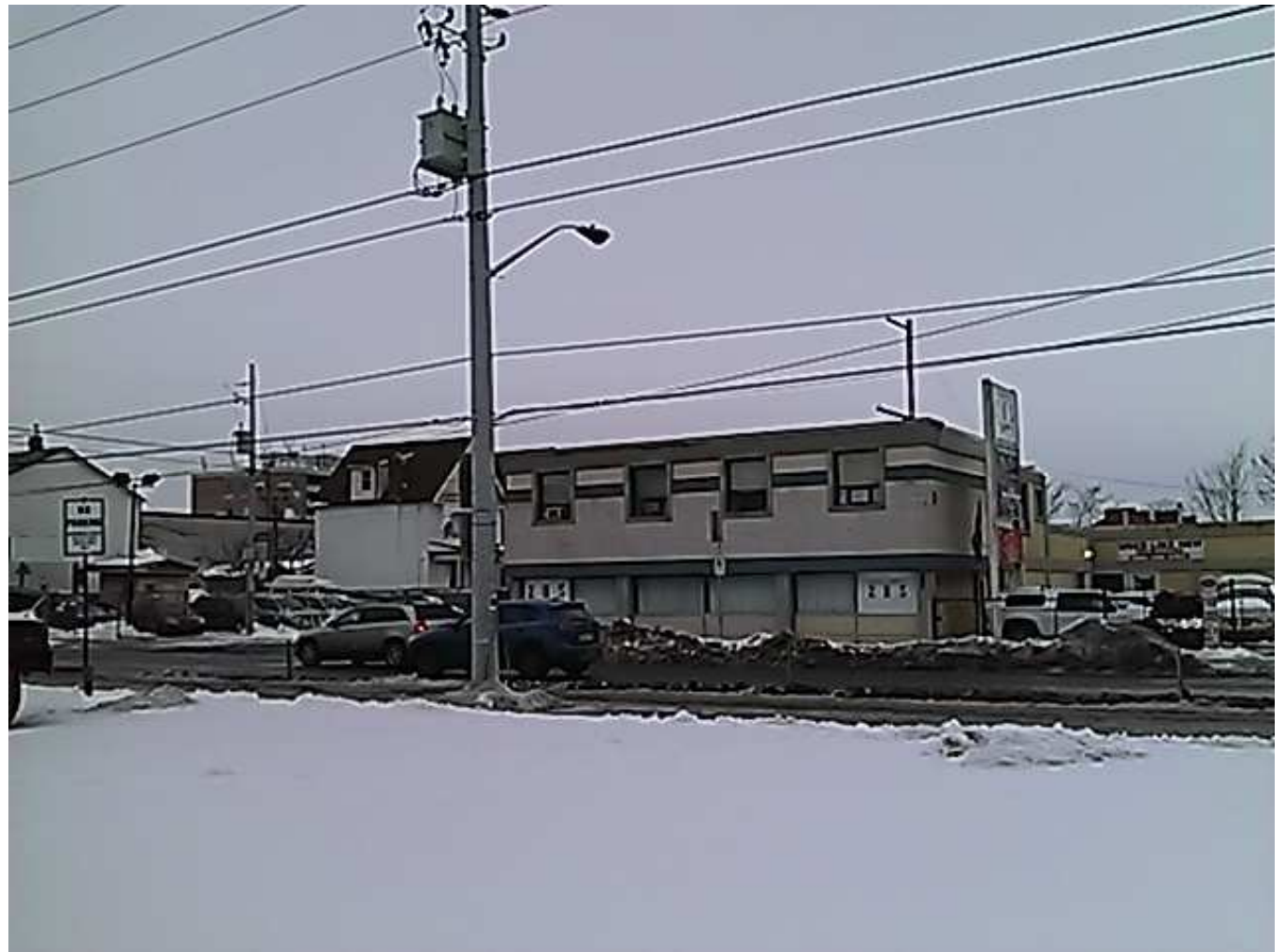
Photo 5 – View North across Cannon Street East.
