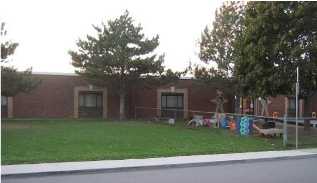
View of 1980s addition (east façade).
