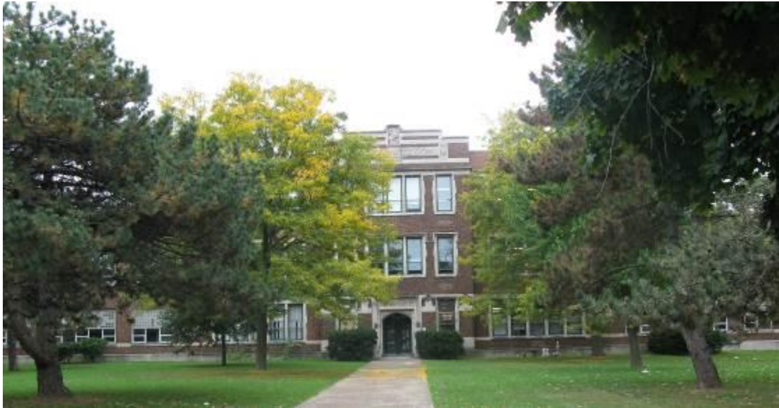
Front (north) façade looking south from Concession Street.
