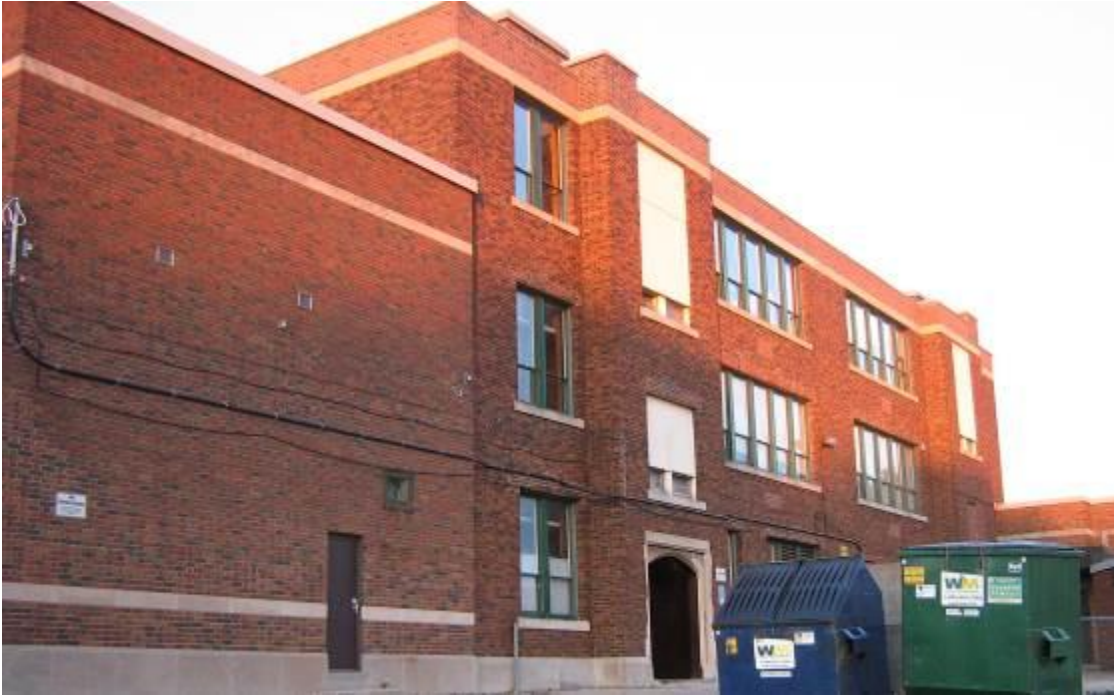
Rear (south) façade looking northeast from East 18 th Street.
