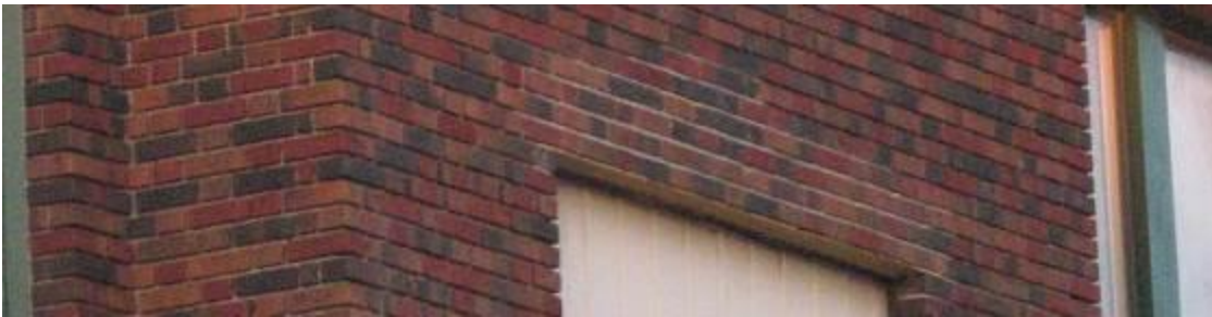
Repointing above rear windows on original portion of school.
