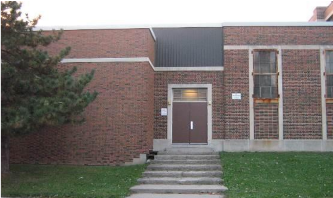
Transition between 1953 addition (right) to 1980s addition (left).
