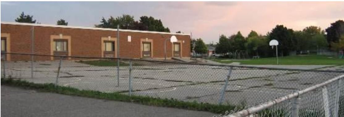
View of rear school yard looking southeast from East 18 th Street.
