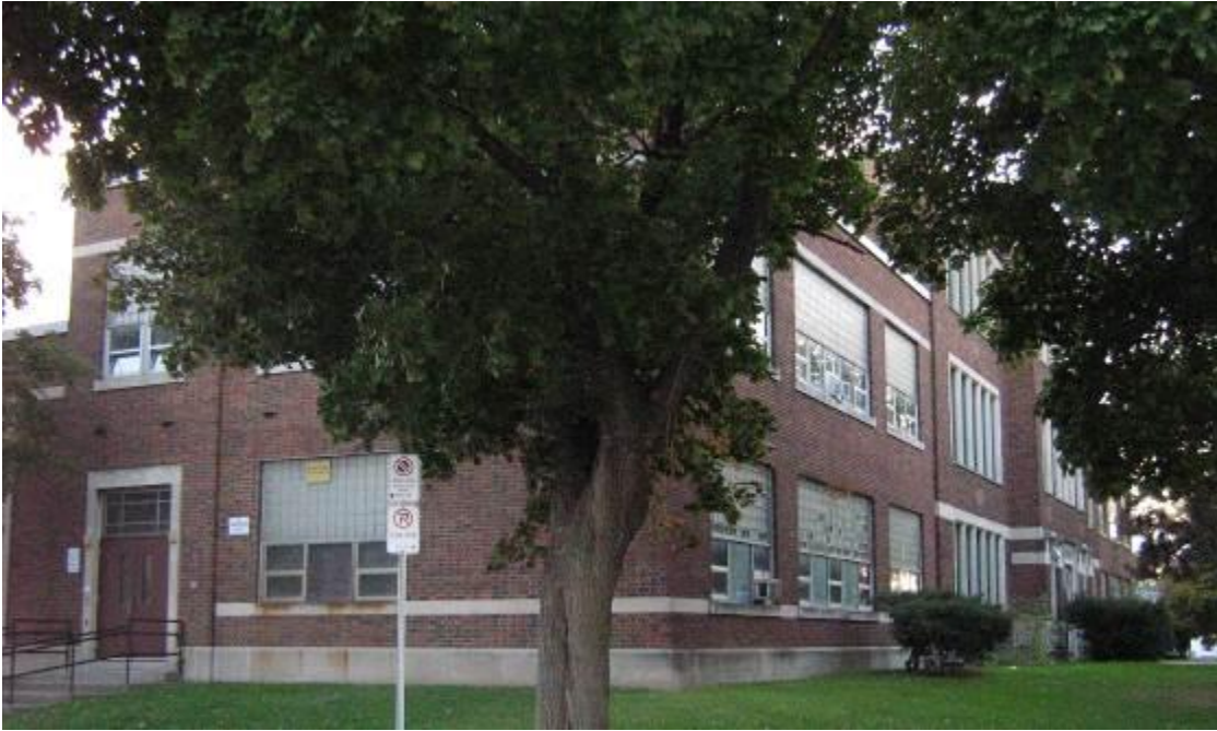
Transition between original portion (far right, three storeys) and 1953 addition (left).
