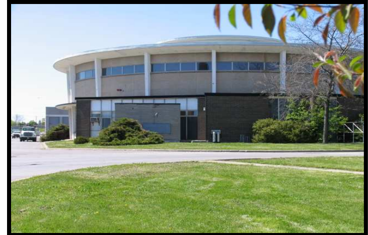
Main Pump House
