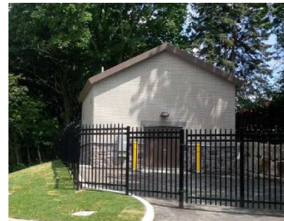
Old Ancaster Rd Water PS Substantial Performance 2015
