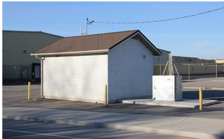
Real Time Control – Burlington St & Wellington St
