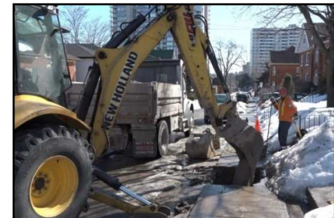
Water Service Thawing
