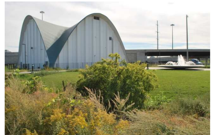
Low Lift Pumping Station
