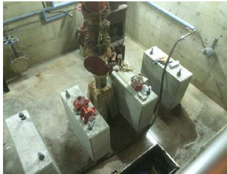
Twenty Rd SPS Construction 2015
