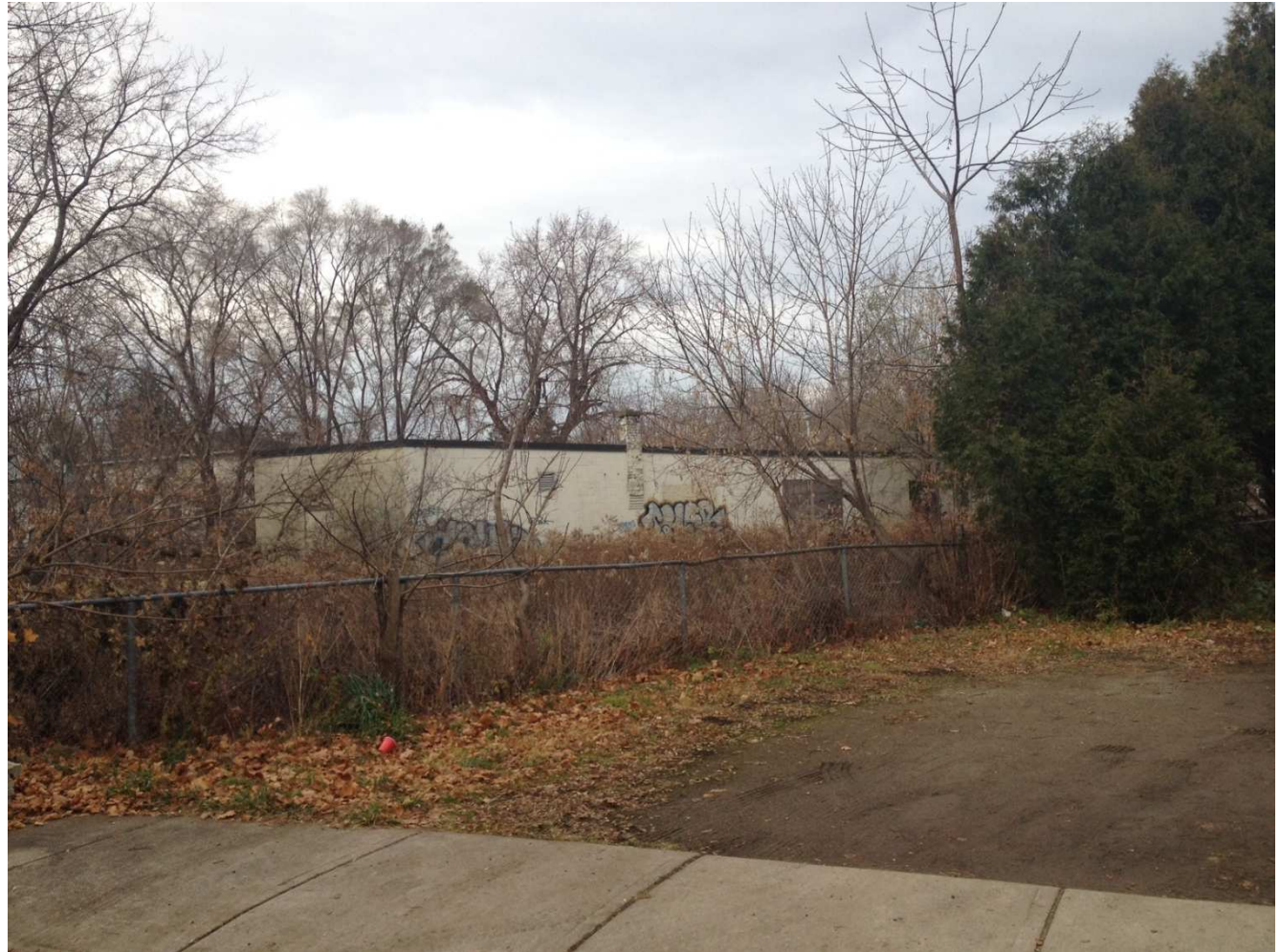
Photo 11 – Rear of Subject Lands – View from Aylett Street.
