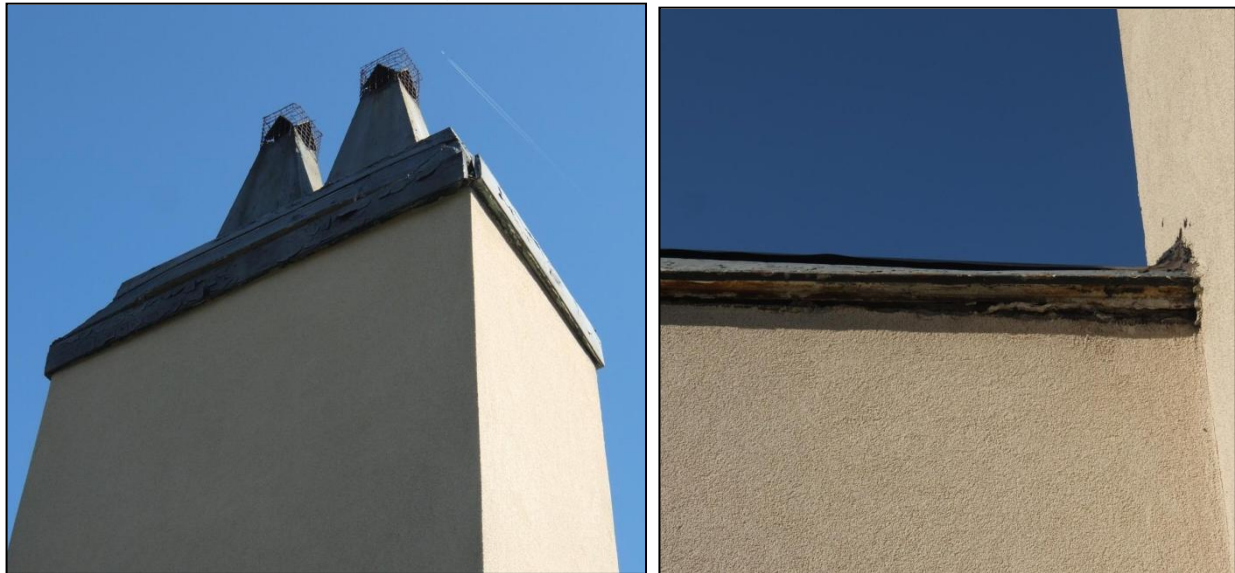
Typical chimney and roof flashing condition (October 2015)
