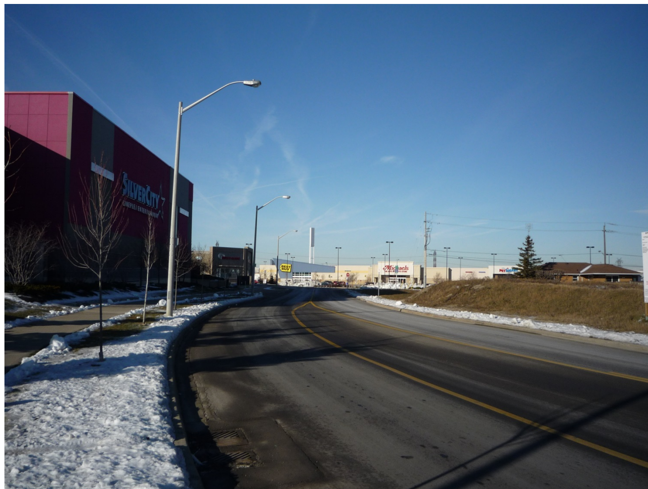
Photo 3 – View West along Artfrank Drive.
