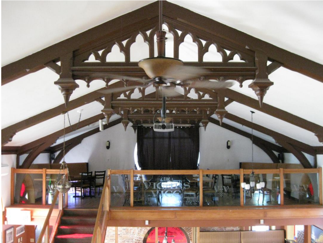
2251 Rymal Road East, Stoney Creek – Interior View, looking towards front of the building and the balcony (2015)
