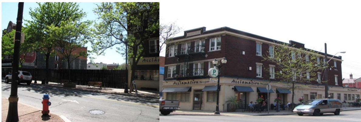
179-191 James Street North in its existing condition
