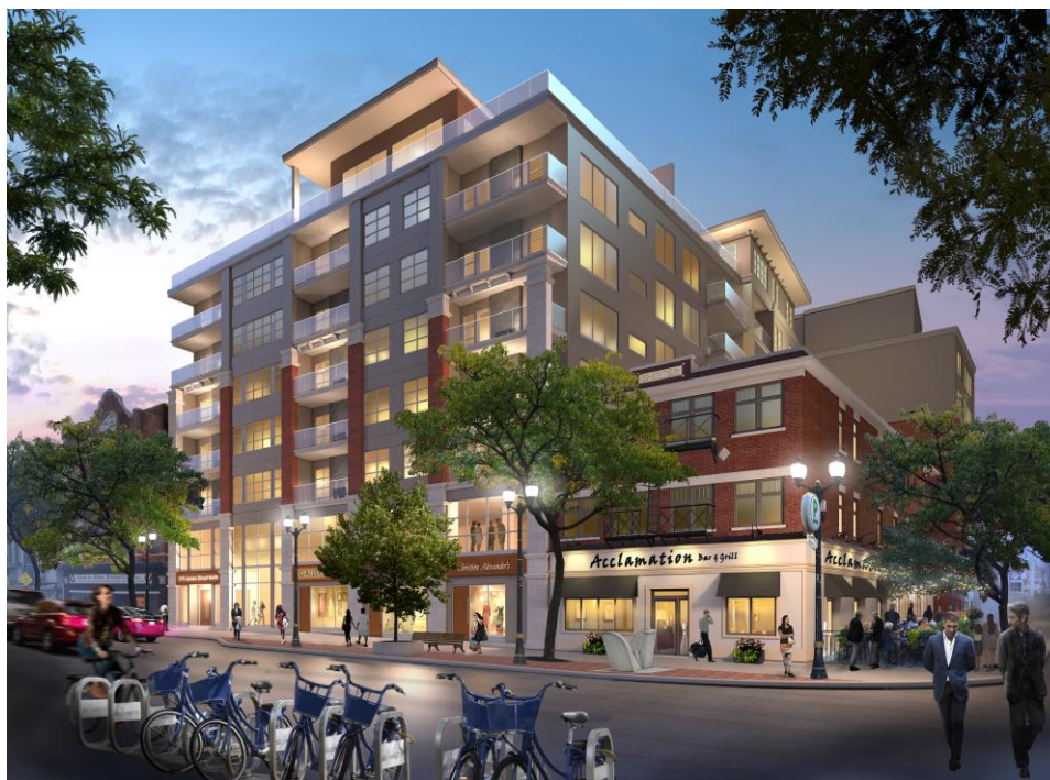
179-191 James Street North post-development
