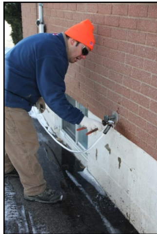
House to House Connections
