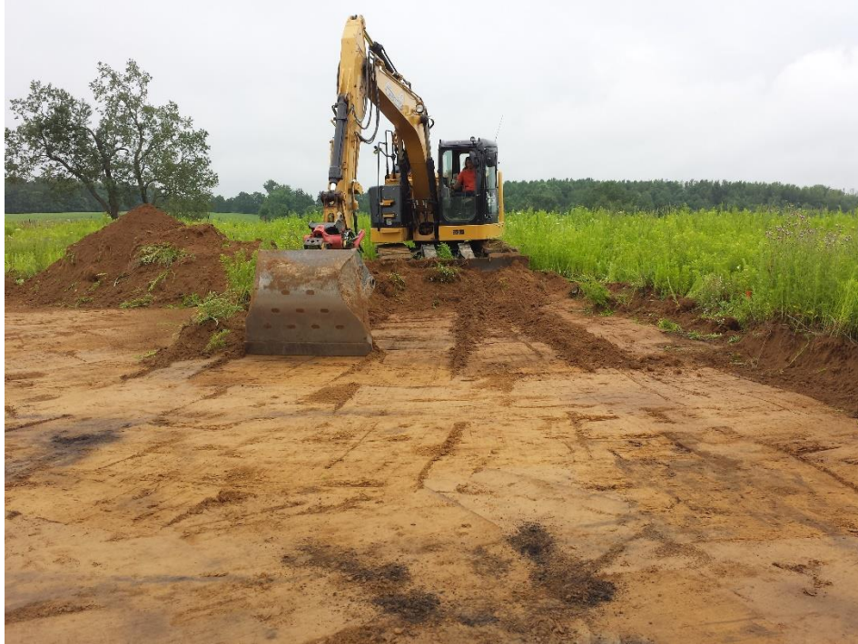
Image 5: Mechanical Topsoil Removal in Progress. Facing South.
