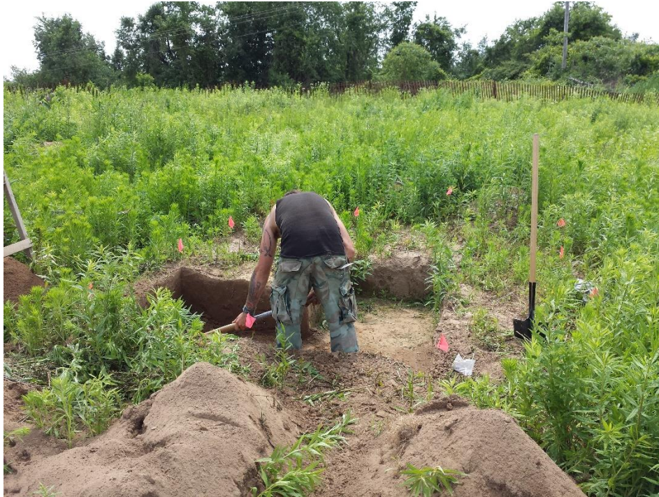
Image 3: Excavations in Progress. Facing West.
