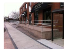
Urban Braille sidewalk, impressed concrete boulevard and accessibility ramp
