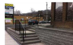
Urban Braille sidewalk, re-constructed retaining walls, stairs and railings
