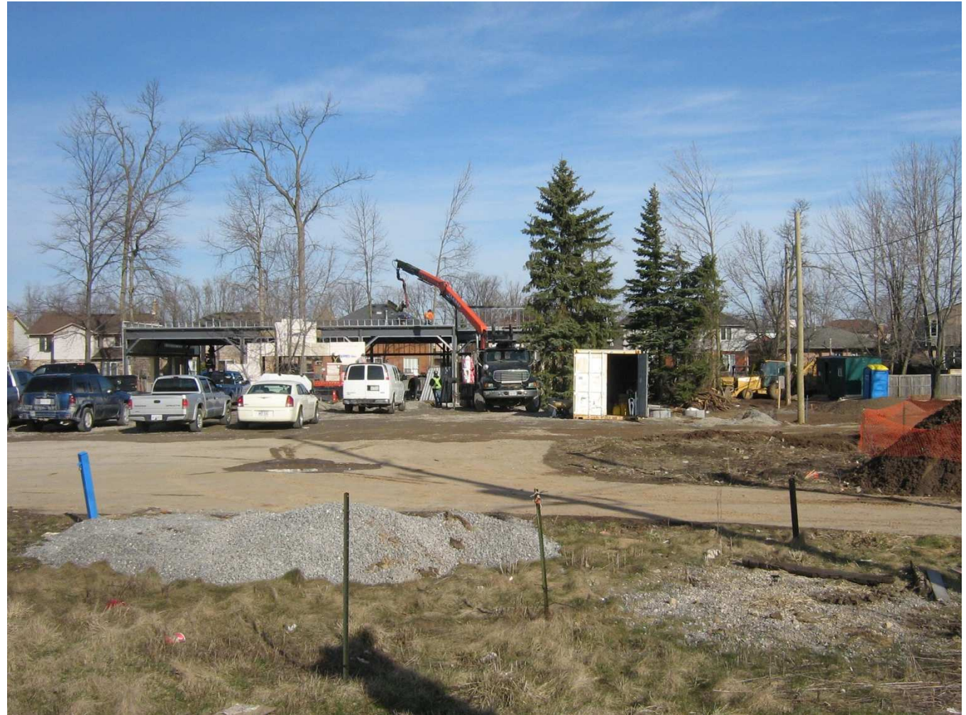
Photo 3 – Construction of daycare facility at 221 Dundas Street East.
