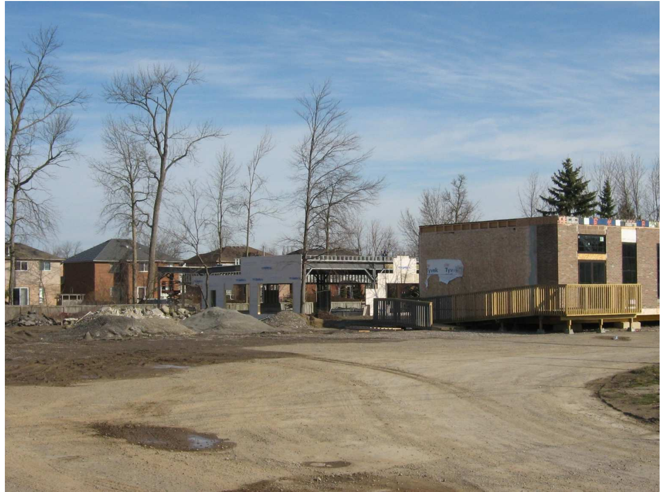
Photo 6 – View looking north through subject site.
