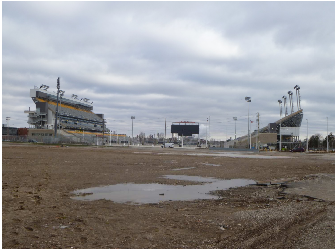
Photo 3 – Current view north from King Street East, across the South Stadium Precinct to Tim Horton’s Field.
