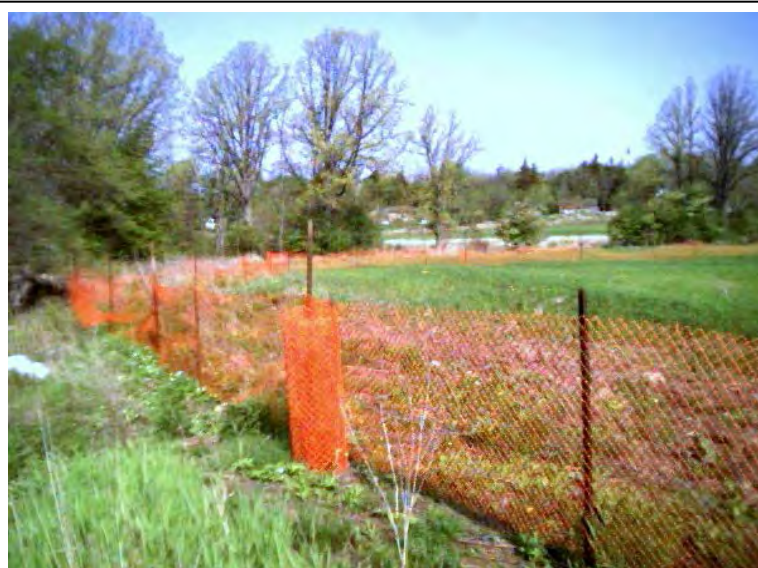
Temporary snow-fencing is erected to establish a buffer area of 20 meters surrounding an identified archaeological site, to temporarily protect it from disturbance by construction activities on adjacent lands, until permanent protection is put in place.
