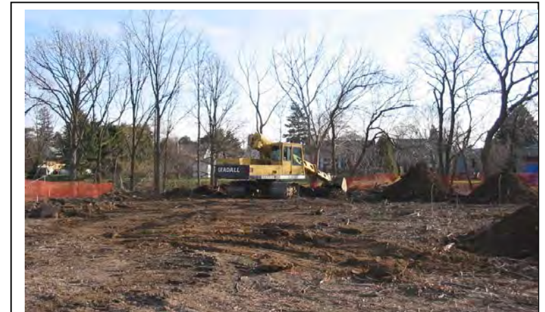
Under direction of an archaeologist, a Gradall with a ‘toothless’ bucket is being used to mechanically strip topsoil from a site. The last few centimetres of topsoil are removed manually by shovel, to clean the top of the subsoil surface and expose any cultural features present( ‘shovel-shining’). They can then be mapped, excavated and recorded. (Image courtesy of Archaeological Services Inc.)
