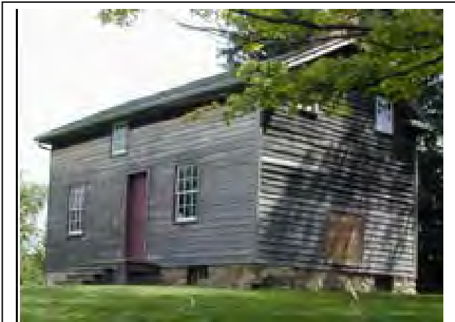
Griffin House in Ancaster is an early African-Canadian farmstead associated with refugees from the United States that arrived via the underground railway. Such properties may yield potential archaeological artifacts related to these early pioneer activities.
