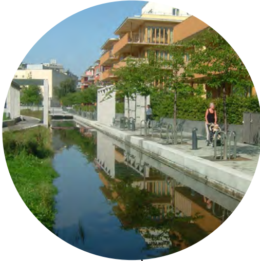
A Pedestrian and Cyclist Greenway that captures stormwater and provides an east-west connection
