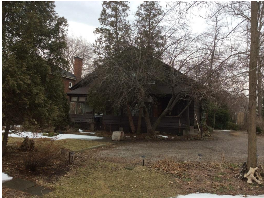
Photo 2 - View of Rear of Dwelling
