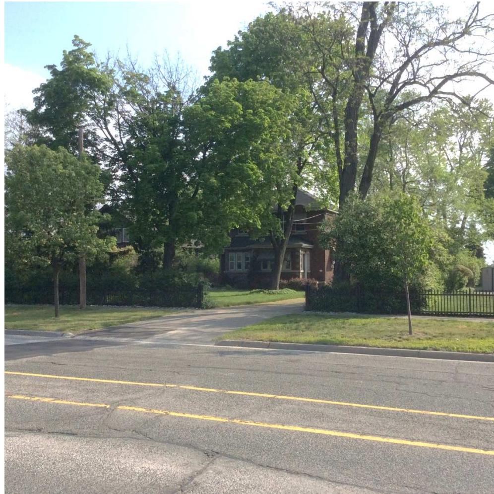
Photo 6 – Adjacent dwelling at 267 Beach Boulevard.
