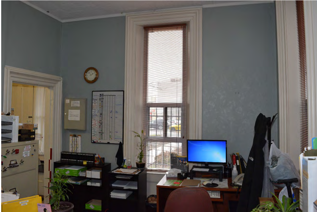
Figure 46: Door and window surrounds in the southeast room.
