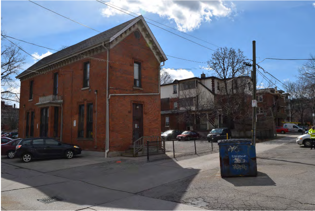
Figure 15: View facing southeast showing the west side of the Study Area.
