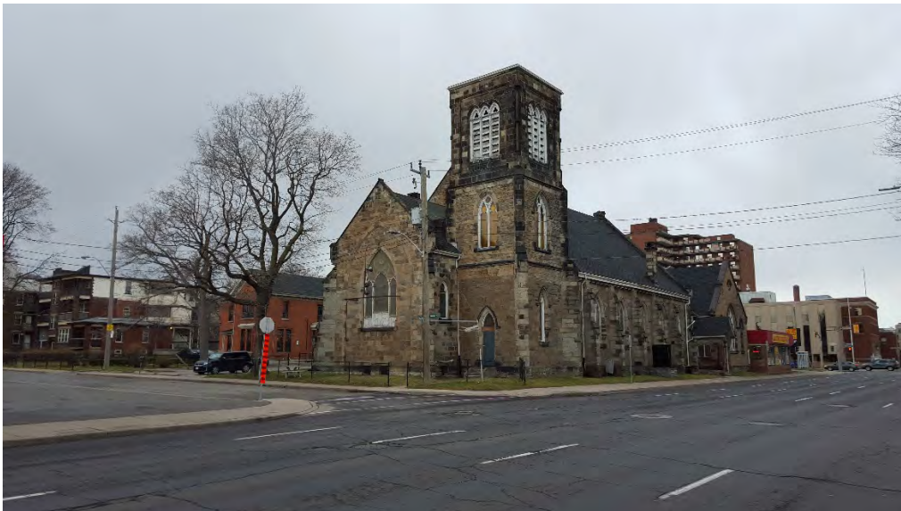
Figure 20: View facing southwest of the Church of St. Thomas and the Parsonage from approximately the same location as the 1890s photograph (Figure 6).
