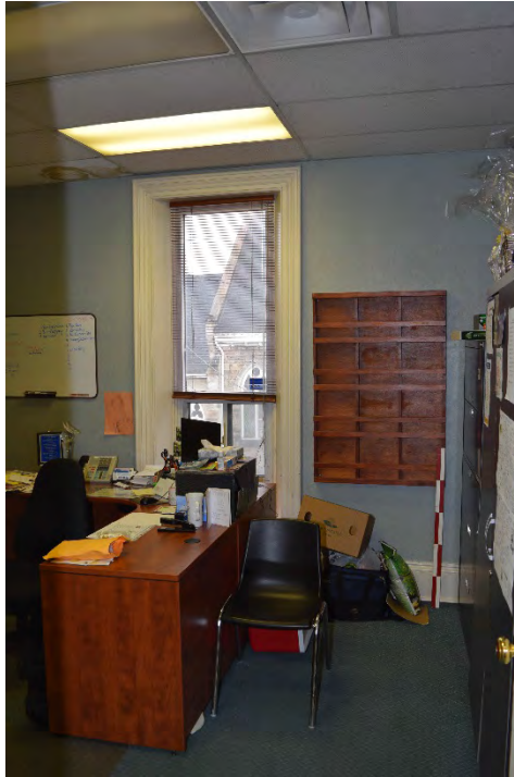
Figure 48: Hanging ceiling, window surrounds and baseboard on the second level.
