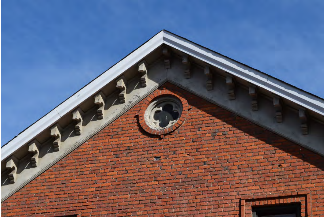
Figure 34: View of the oculus and quatrefoil window on the south gable.
