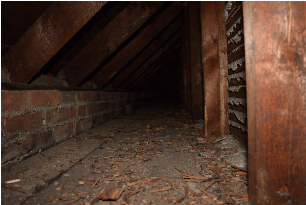
Figure 53: View of the top of the wall, rafters, and lathe-and-plaster through the small access hole.
