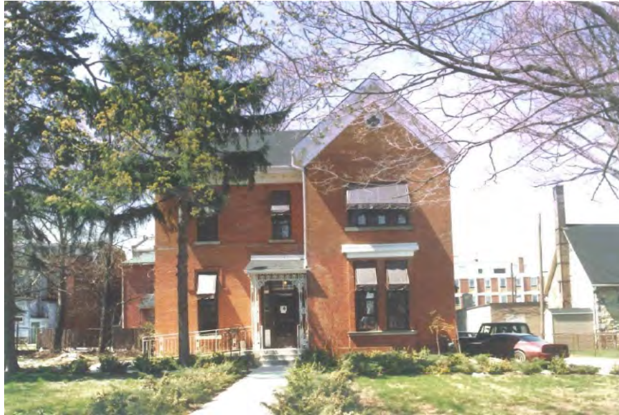
Figure 12: 1991 file photograph of the Parsonage (courtesy City of Hamilton).
