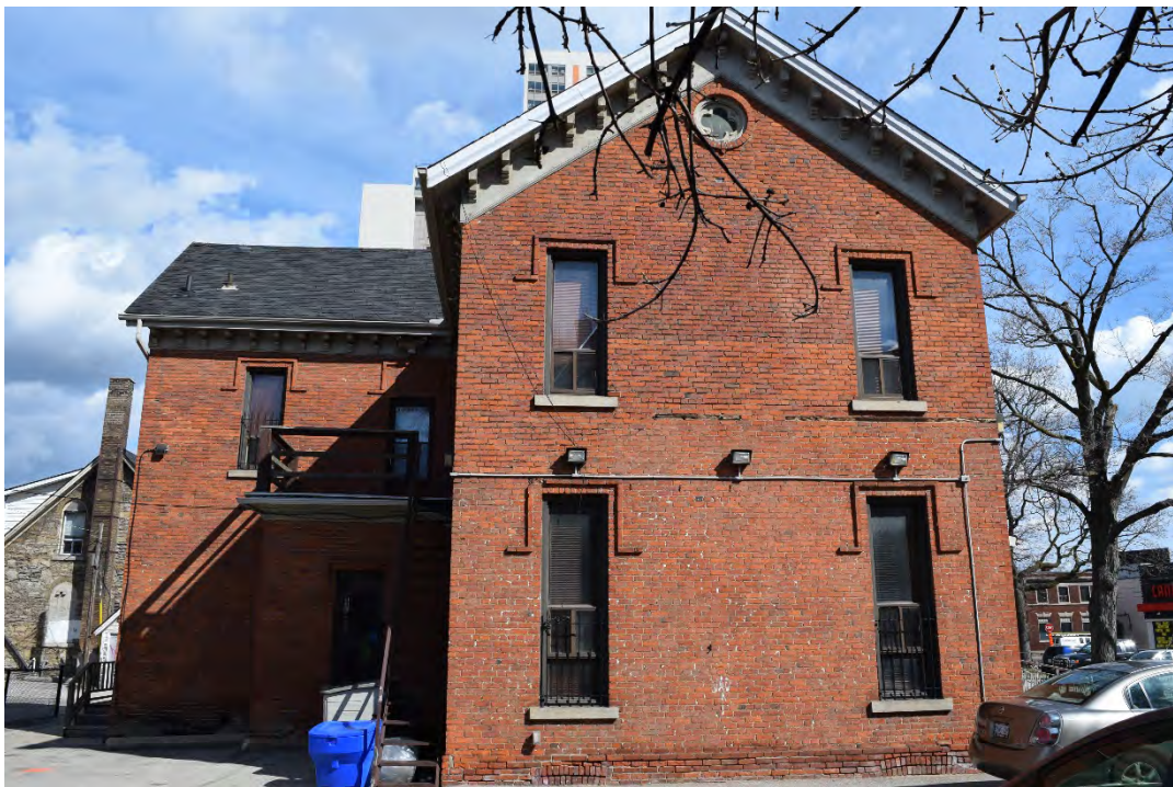
Figure 23: The south façade of the Parsonage.
