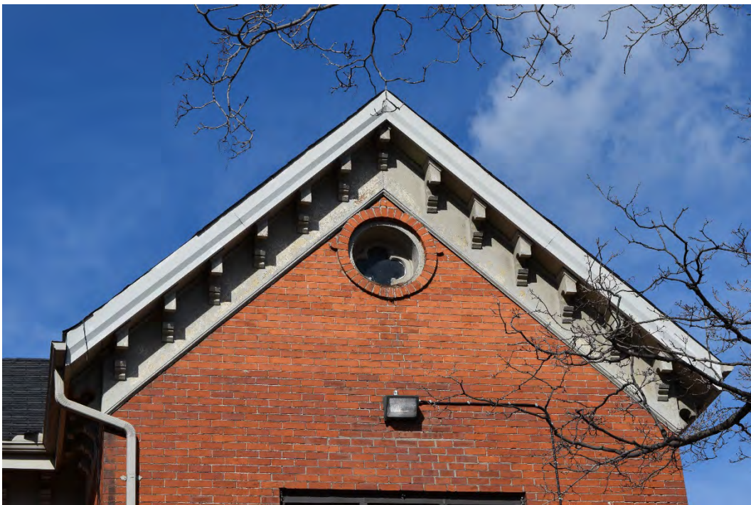
Figure 29: View of the east gable showing the frieze and brackets.
