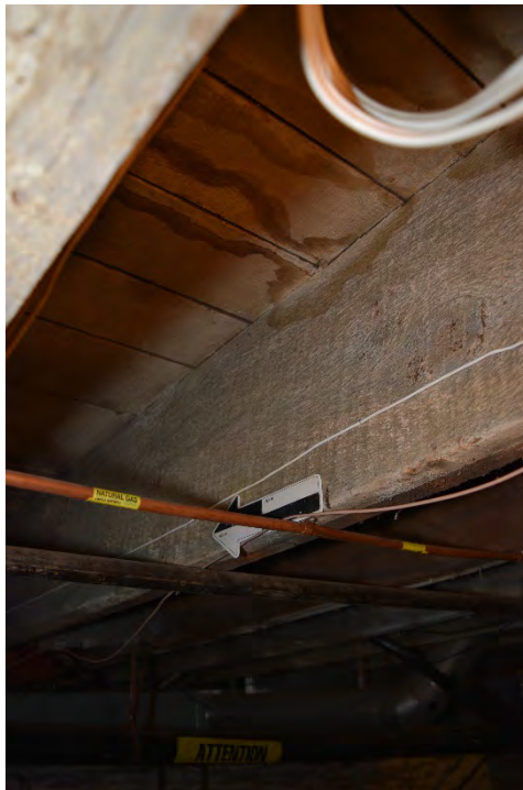
Figure 41: Circular saw marks are visible on the joists.
