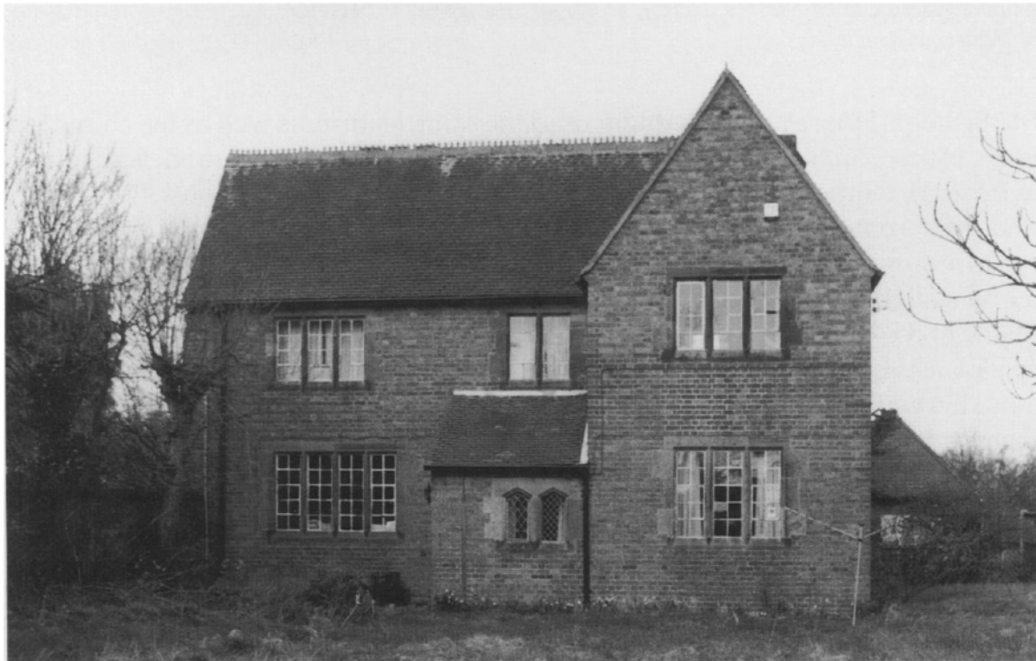
Figure 54: A presbytery designed by Pugin with similar features to the Parsonage, including construction in brick, orientation of the T-plan, central entrance, and the combined windows (from Hill 2003:159).
