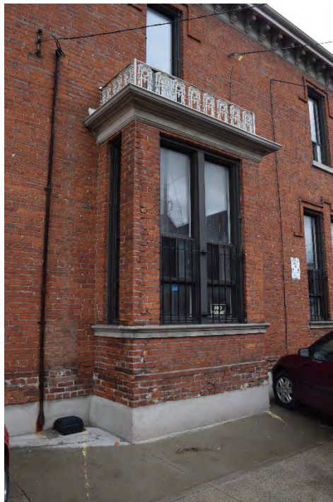
Figure 33: The north projecting bay, facing southwest.
