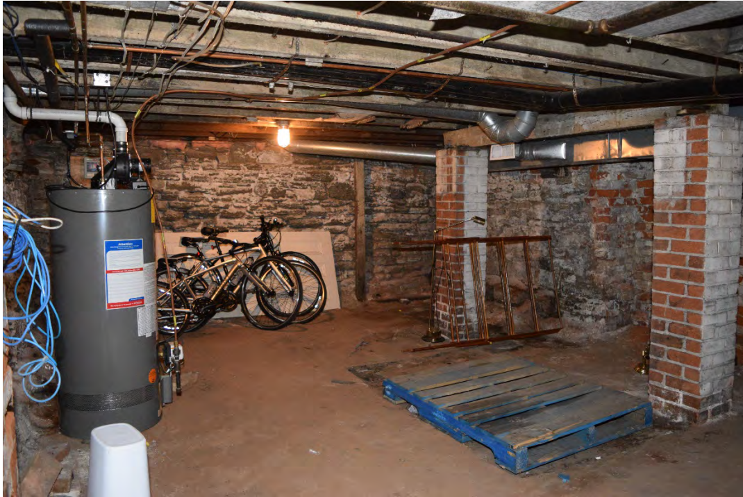
Figure 40: The southeast corner of the basement in the north section.
