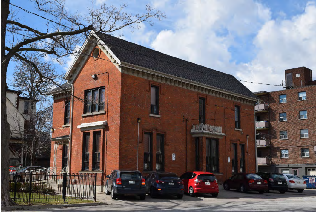
Figure 26: East and north façades of the Parsonage.
