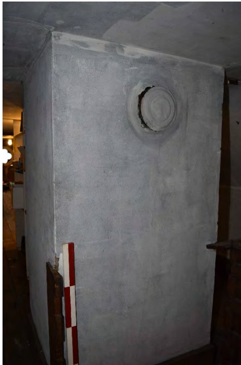
Figure 52: The chimney base in the north section attic.
