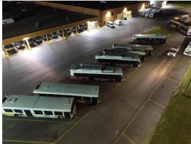
Figure 1 – 2200 Upper James, rear (west) of MSF showing full garage and outdoor storage
