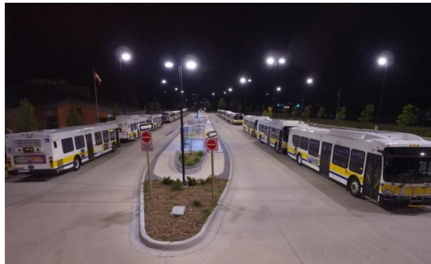
Figure 2 – 2200 Upper James, front (east) of MSF showing outdoor storage within the Park and Ride terminal
