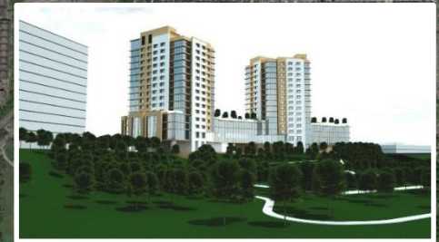
CIC Project – 925 Main Street W
