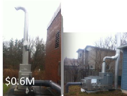
Carbon Filters: Beach Blvd & Upper James Substantial Performance 2016
