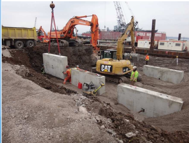
Anchor Block Lowered into position
