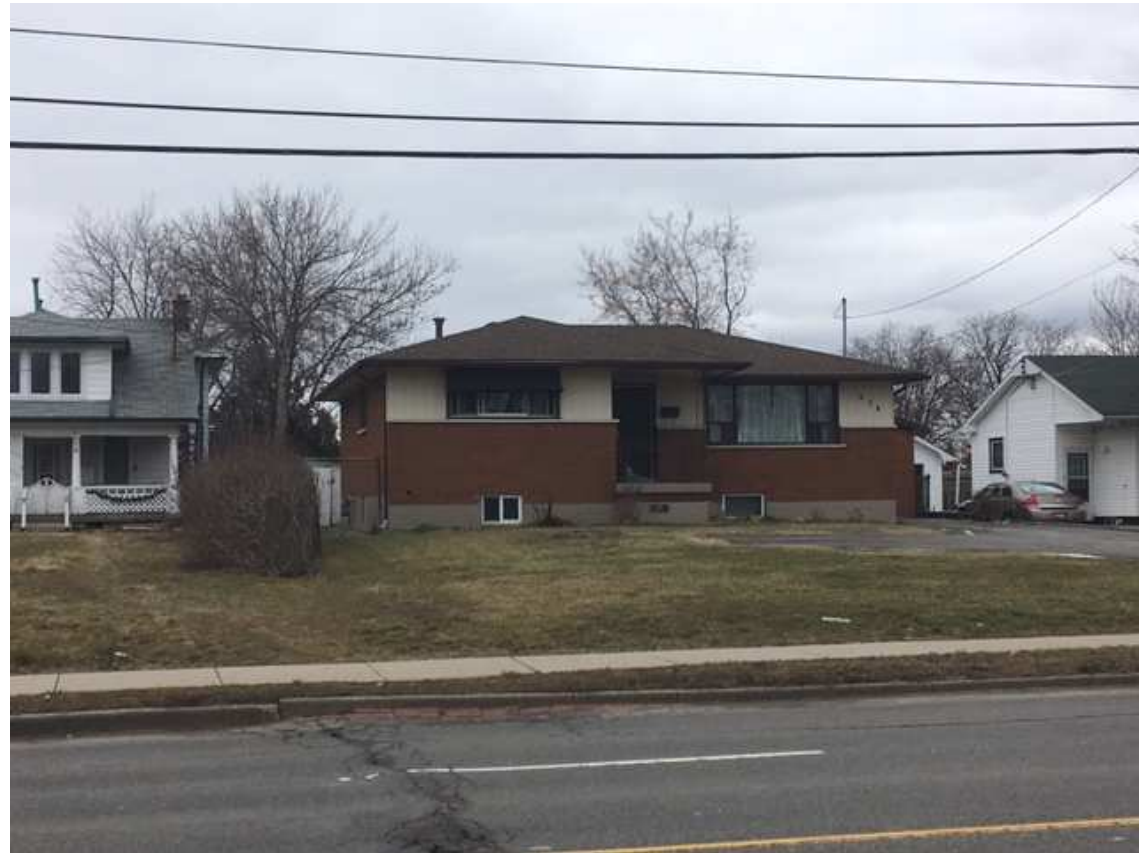
Photo 4 – 938 Upper Gage Avenue – Lands to the North of the Subject Lands
