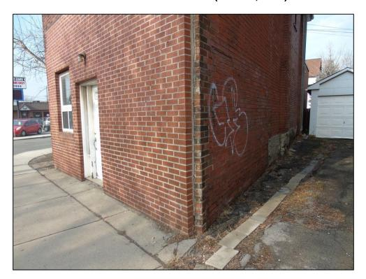
Photograph 4: View showing detail of the corner of 1137 King Street East. The addition can be seen joining the original structure at right where the foundation changes (AECOM, 2017)
