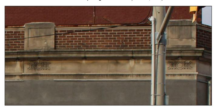
Photograph 4: View showing motifs located below the concrete panels in the parapet wall. It is likely that below these motifs, pilasters divided the façade into bays to articulate a formal composition (AECOM, 2017)
