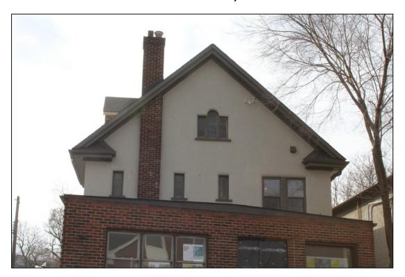
Photograph 8: View showing detail of windows on north facade of the dwelling, including small Palladian window (AECOM, 2017)
