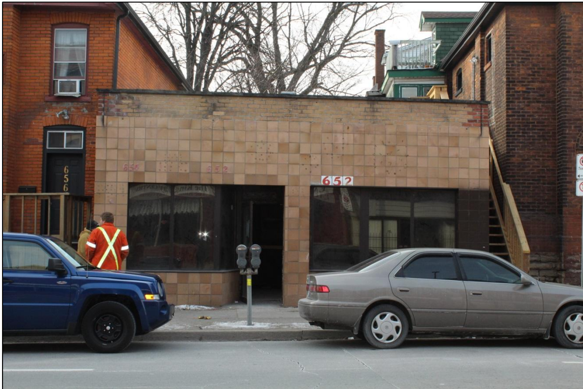
Photograph 1: Façade of 652-654 King Street East (AECOM, 2017)
