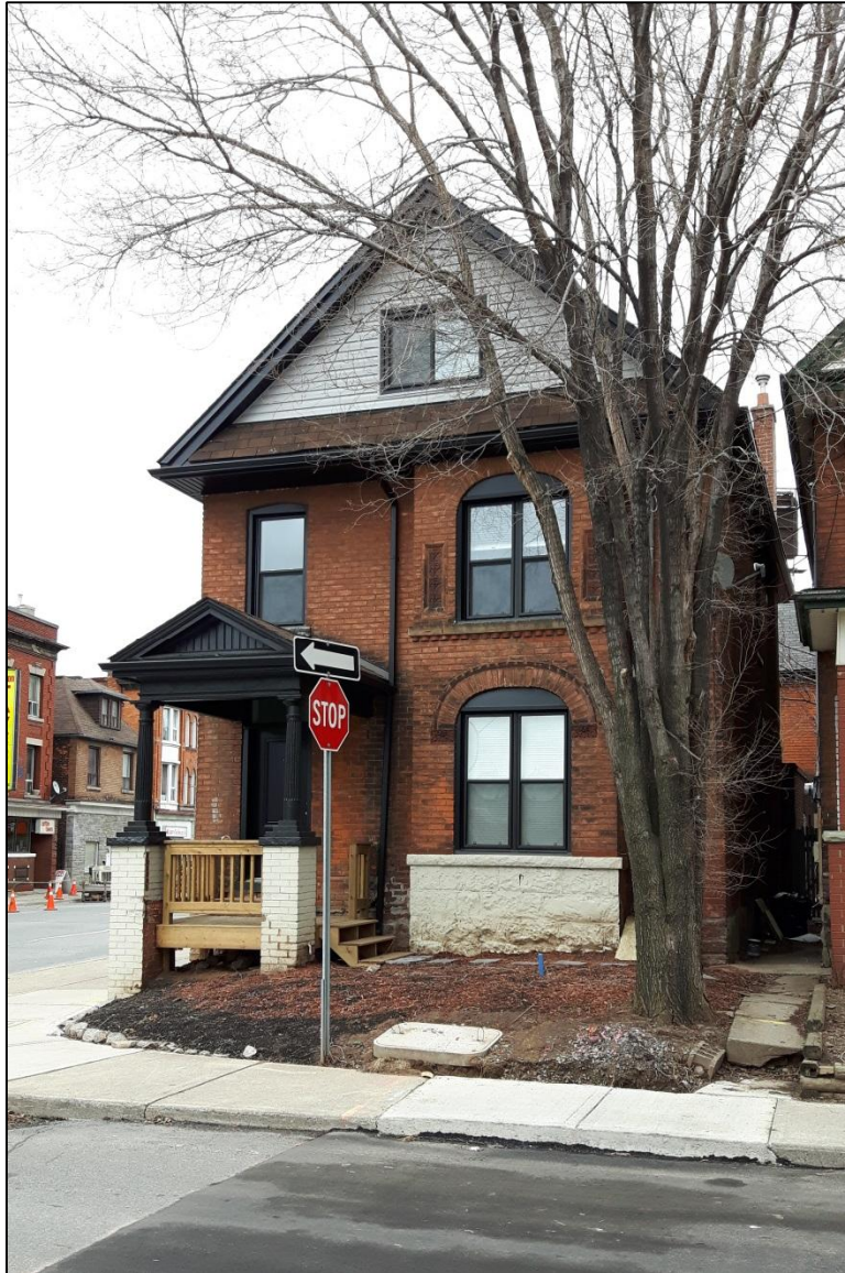
Photograph 2: Façade of 1 Grant Avenue (AECOM, 2017)
