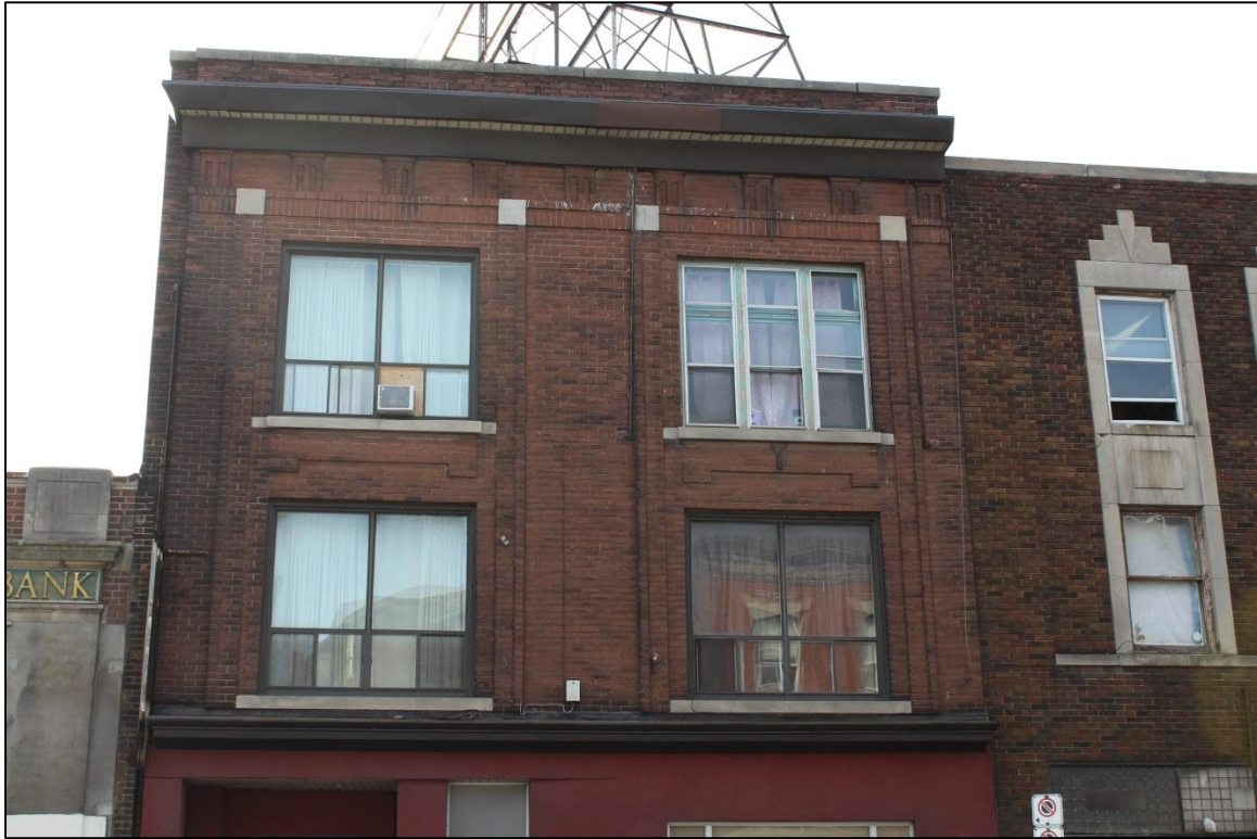
Photograph 3: Second floor of 662 King Street East (AECOM, 2017)
