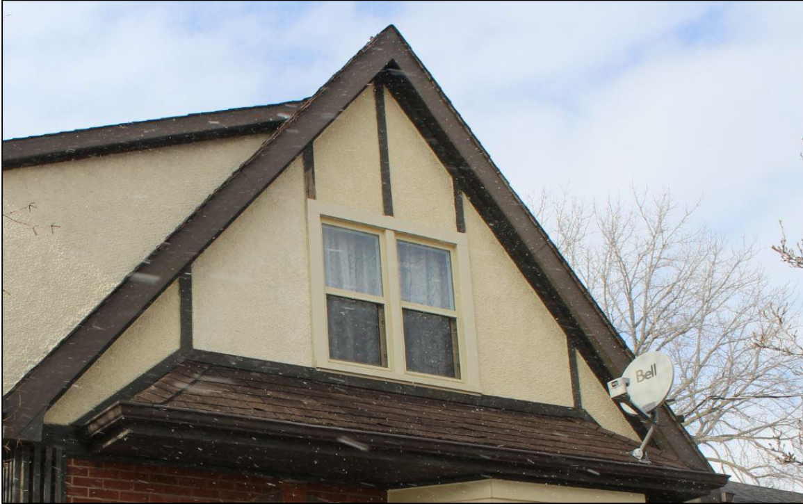
Photograph 5: Detail showing gable peak, upper half-storey windows, bellcast porch roof, and half timbering (AECOM, 2017)
