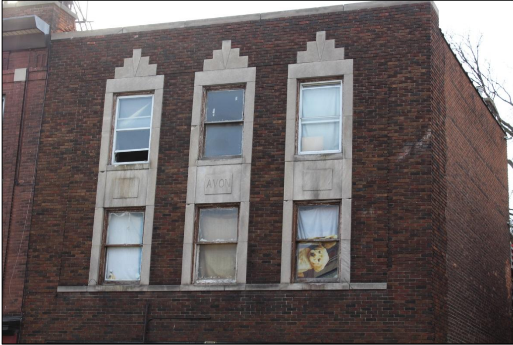
Photograph 4: View showing Art Deco details including concrete panels, surrounds and voussoir designs above windows
