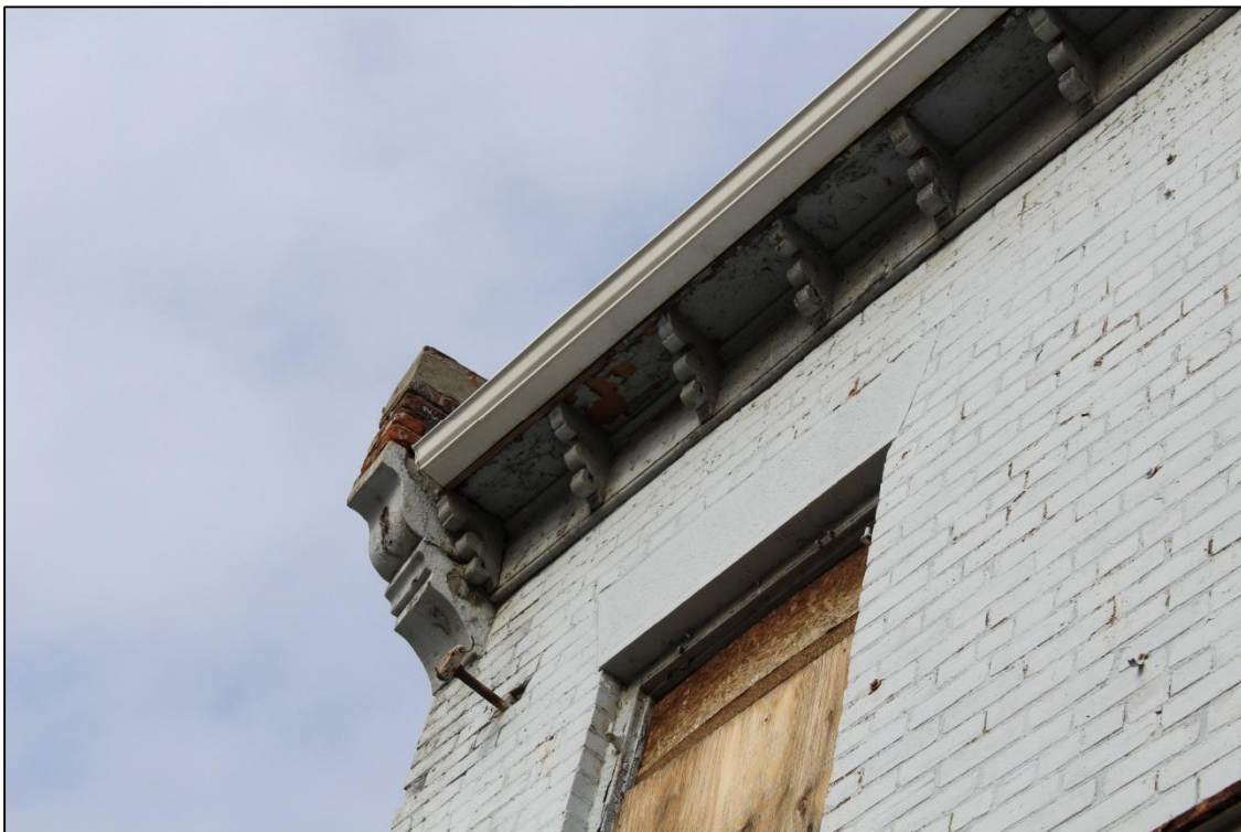
Photograph 6: View showing cornice and bracket details at roofline (AECOM, 2017)
