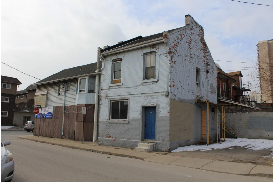
Photograph 7: View showing rear portion of 563 building, formerly 3 Steven Street (AECOM, 2017)
