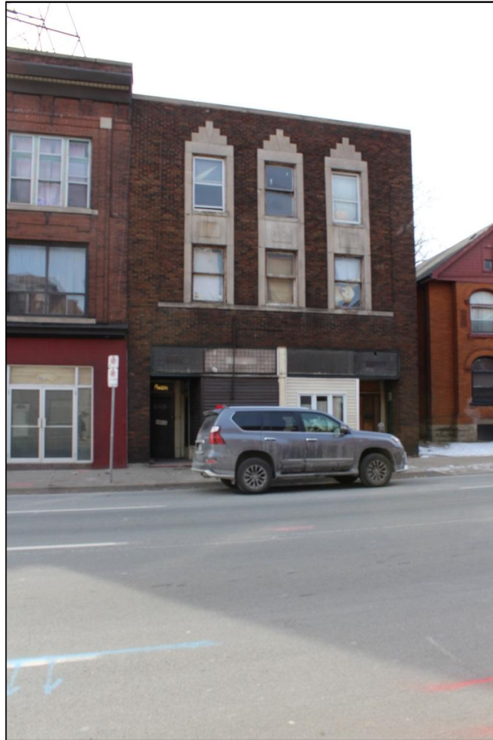
Photograph 1: View looking south showing 658-660 King Street East
