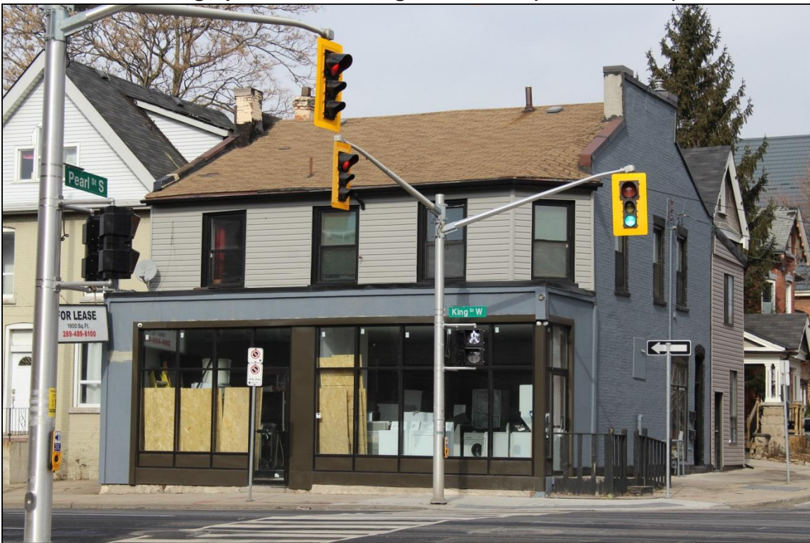
Photograph 2: Façade of 426-428 King Street West (AECOM, 2017)
