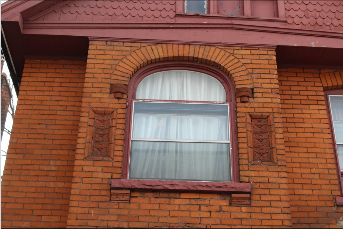
Photograph 3: Details fielded panels and basket arches articulated by an edging around the voussoirs and decorative moulded terracotta labels and bracket on the second floor of 656 King Street East (AECOM, 2017)
