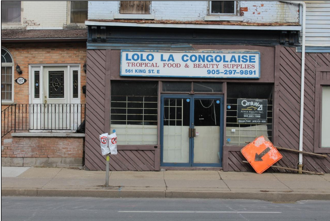
Photograph 3: View showing ground floor details on 559/561 building (AECOM, 2017)
