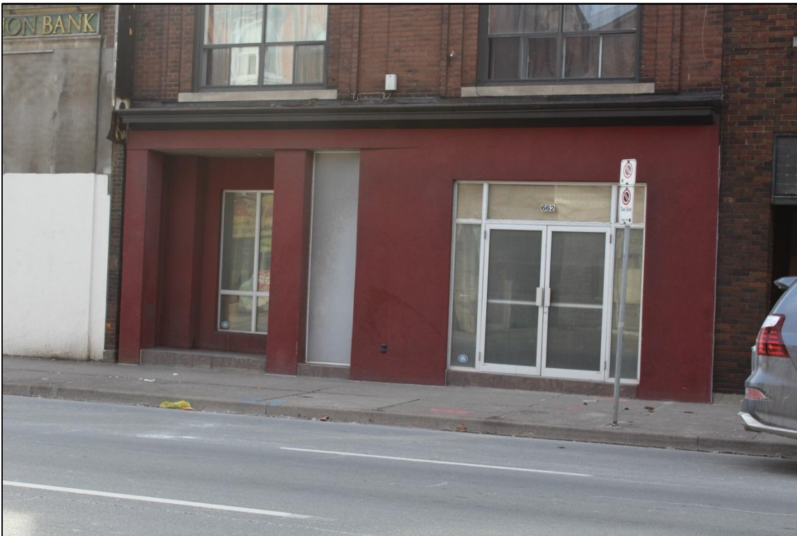
Photograph 2: Main floor of 662 King Street East (AECOM, 2017)
