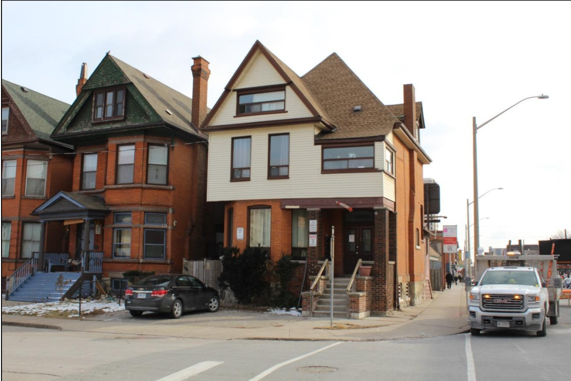
Photograph 1: View to north showing the subject property (right), in relation to similar structures along West Avenue North
