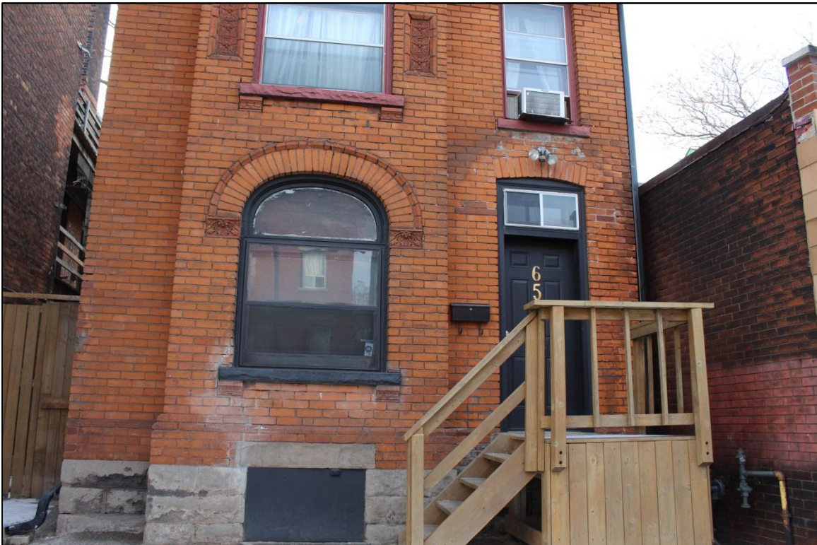
Photograph 2: Details of window sills and basket arches articulated by an edging around the voussoirs on the main floor of 656 King Street East (AECOM, 2017)
