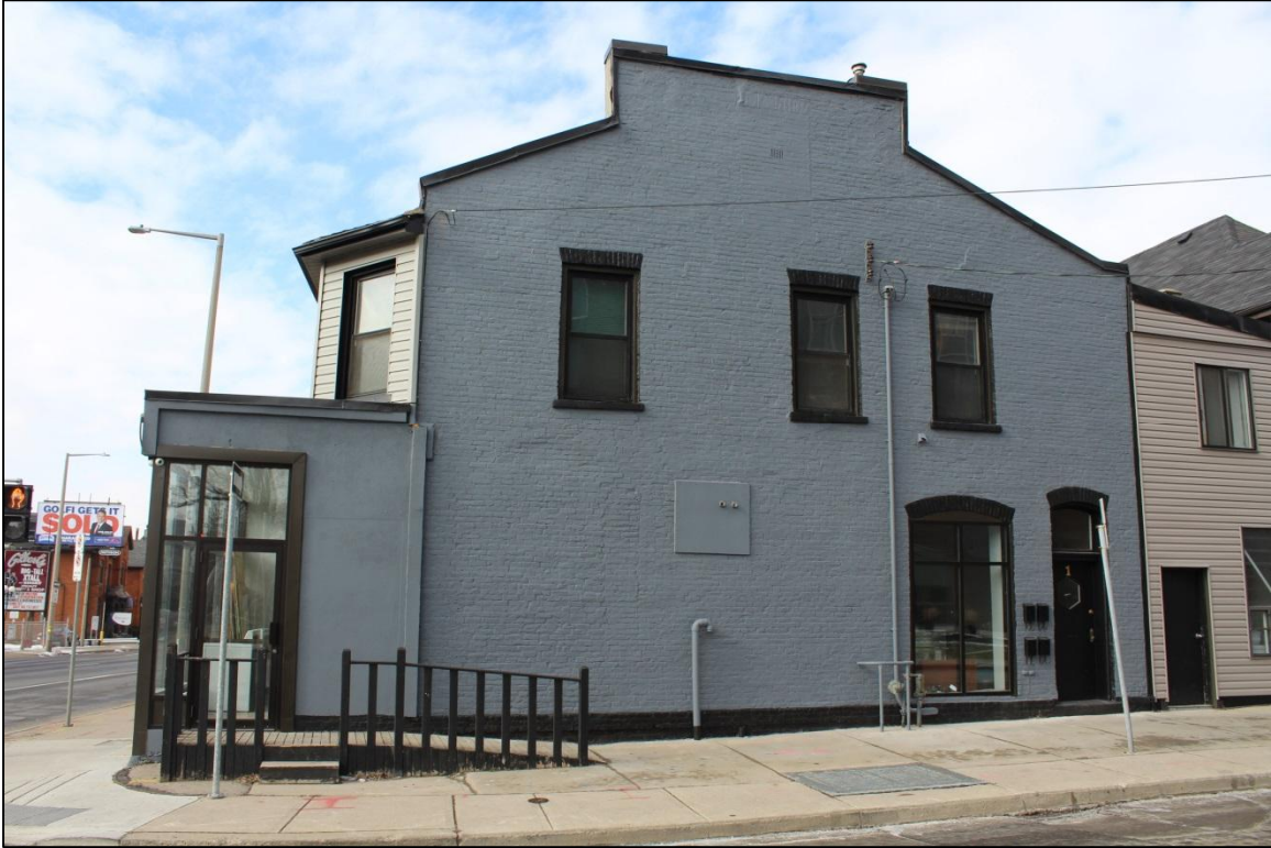
Photograph 3: East-facing façade of 426-428 King Street West (AECOM, 2017)
