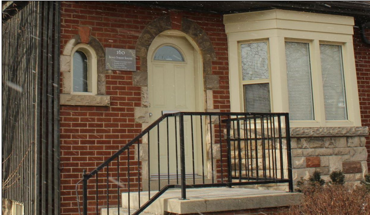
Photograph 4: Detail showing brick exterior and faux stone window and door surrounds, designed to look like masonry voussoirs (AECOM, 2017)
