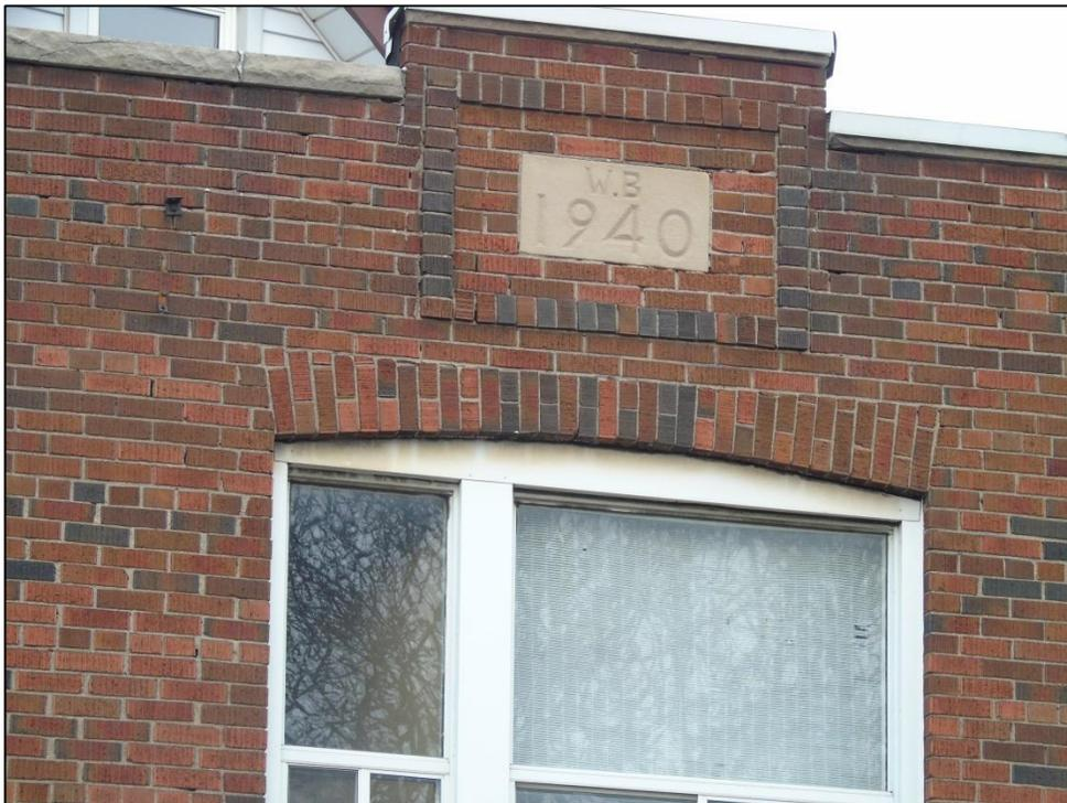
**Photograph 6: View showing detail of raised parapet and concrete/stone panel with "W.B 1940" above second storey window (AECOM, 2017)**
