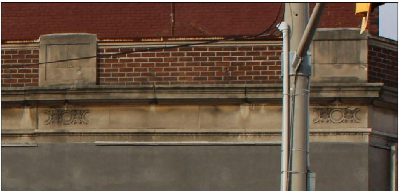
**Photograph 4: View showing motifs located below the concrete panels in the parapet wall. It is likely that below these motifs, pilasters divided the façade into bays to articulate a formal composition (AECOM, 2017)**
