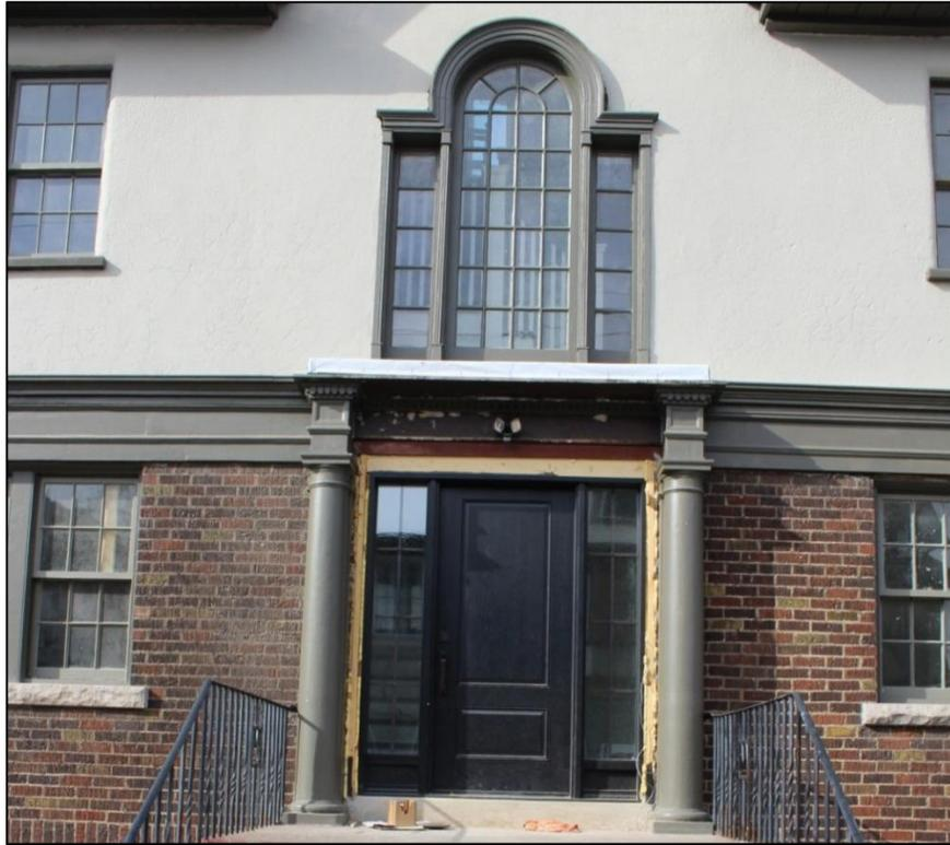
**Photograph 5: View showing detail of centre bay with front door surround and Palladian window above (AECOM, 2017)**
