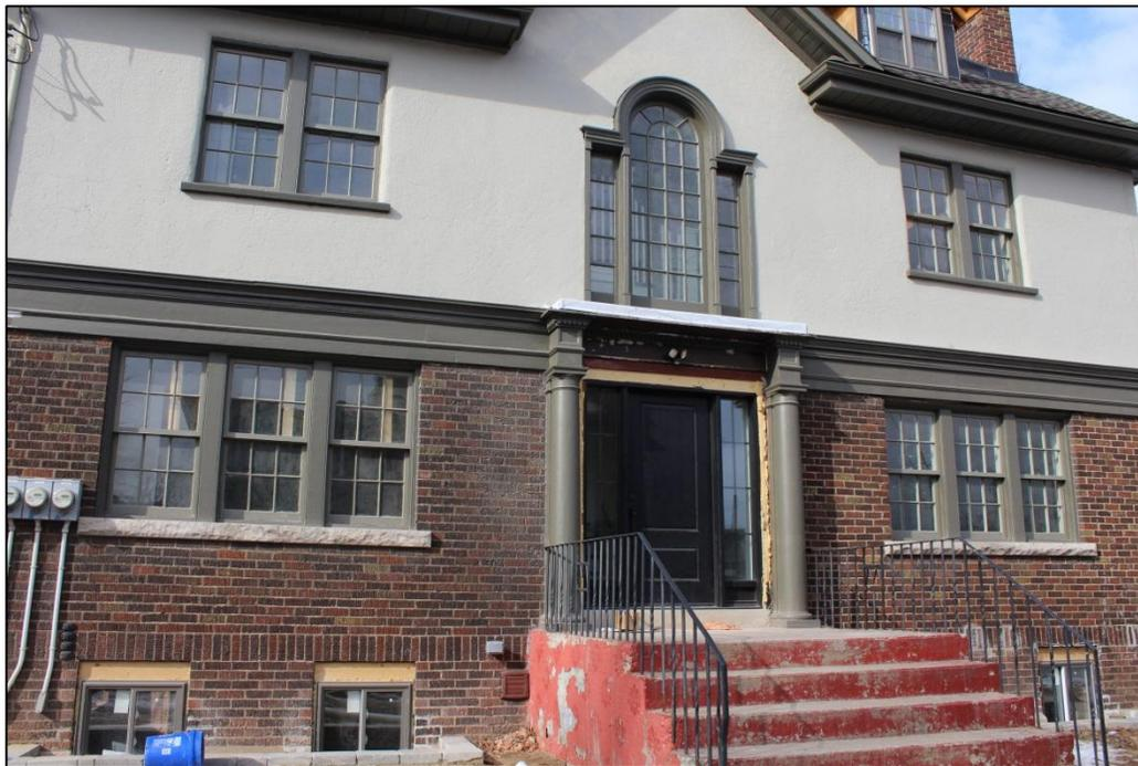
**Photograph 4: View showing detail of three-bay facade and entablature and cornice wrapping around dwelling (AECOM, 2017)**
