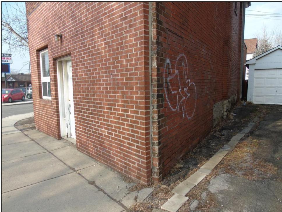
**Photograph 4: View showing detail of the corner of 1137 King Street East. The addition can be seen joining the original structure at right where the foundation changes (AECOM, 2017)**
