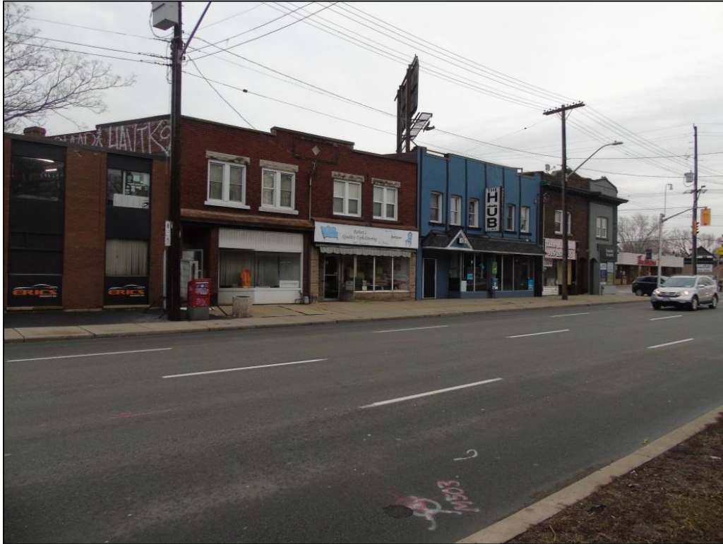
Photograph 1: View looking north showing subject property, second from left in relation to continuous block on King Street East (AECOM, 2017)
