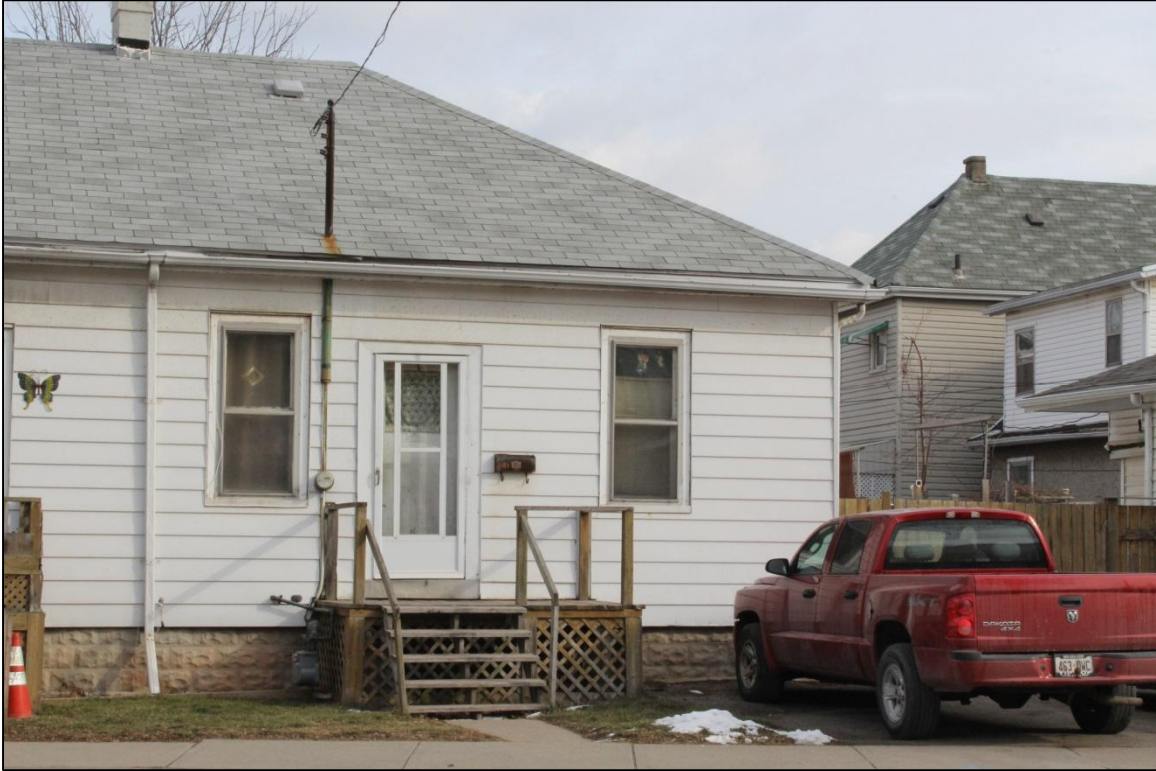
Photograph 3: Façade of 1181 King Street East (AECOM, 2017)
