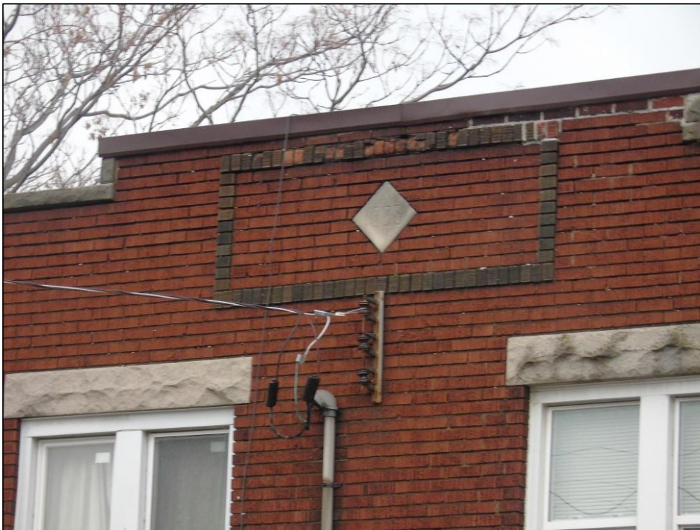
Photograph 4: View showing decorative brick detailing and “1925” concrete date stamp between 1132½ and 1139 King Street East (AECOM, 2017)
