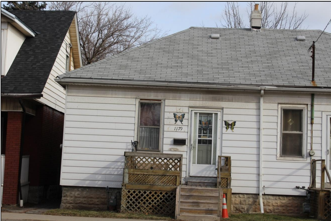
Photograph 2: Façade of 1179 King Street East (AECOM, 2017)
