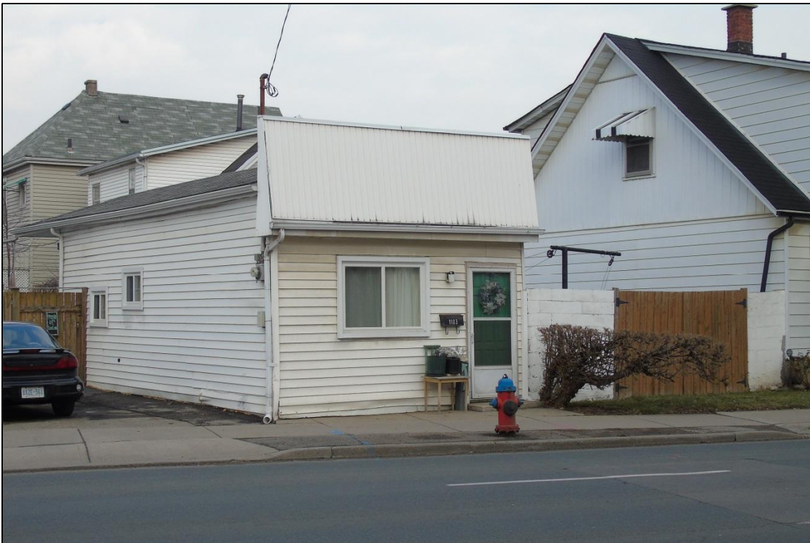
Photograph 2: Façade of 1183 King Street East (AECOM, 2017)
