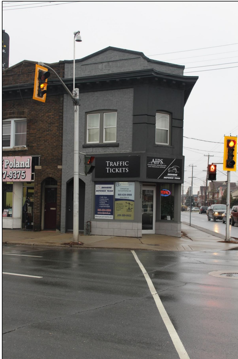
Photograph 5: View looking north across King Street East showing 1149-1151 King Street East (AECOM, 2017)
