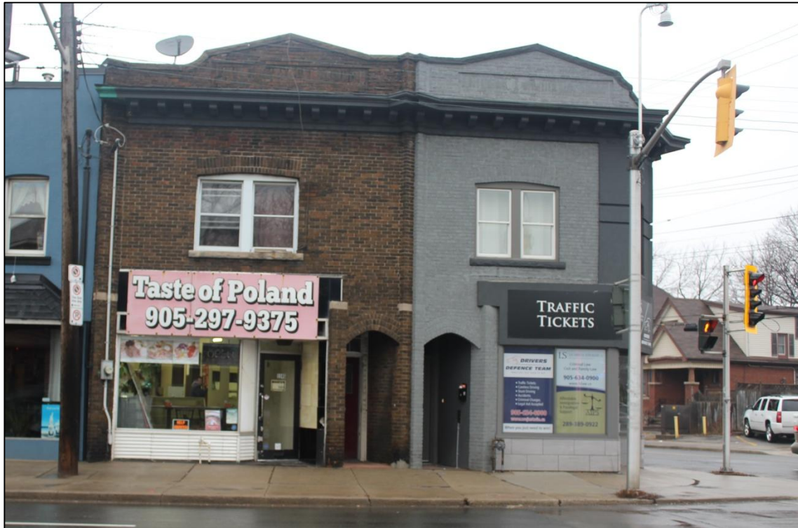
Photograph 3: View looking north along King Street East showing 1145 (left) and 1149-1151 King Street East (right) (AECOM, 2017)
