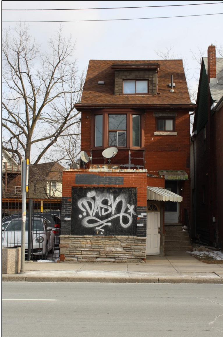
Photograph 1: Façade of 1197 King Street East (AECOM, 2017)
