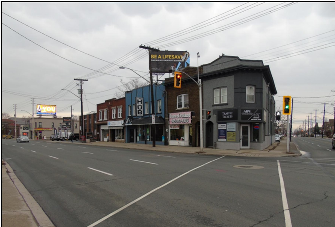
Photograph 4: View looking north across King Street East showing subject property in relation to adjacent building. Intersection at right is Gage Avenue North (AECOM, 2017)
