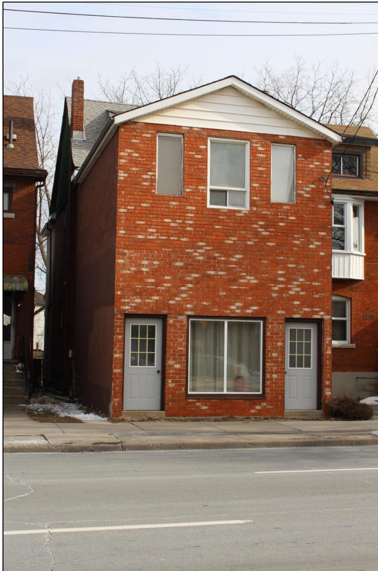
Photograph 2: Façade of 1199 King Street East (AECOM, 2017)
