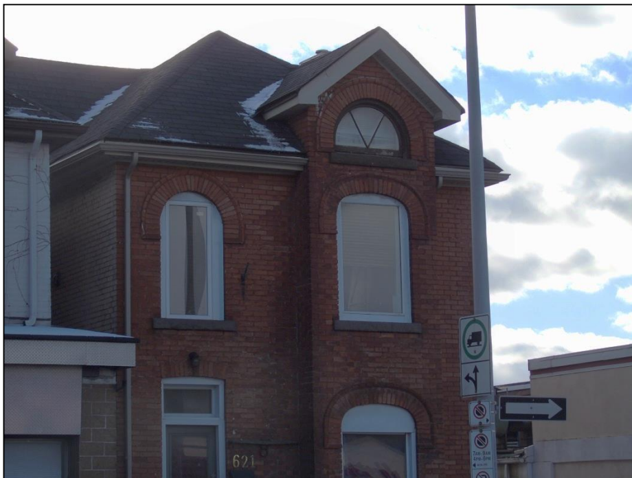
Photograph 6: Details on 621 King Street West, showing similar details to adjacent property and segmental arch lintel above front door transom
