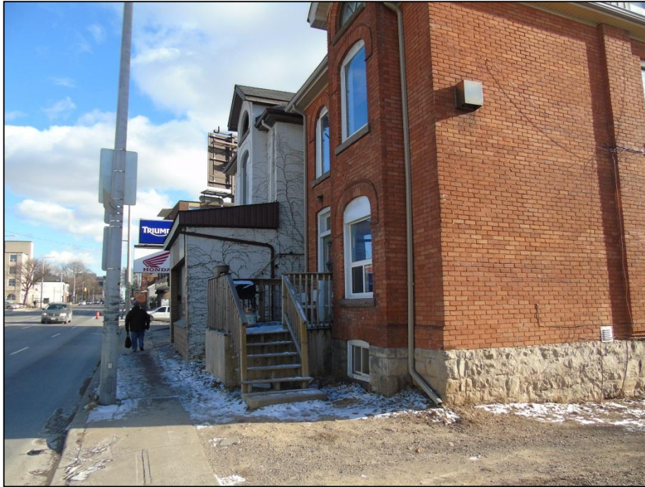
Photograph 3: View looking east showing setbacks of subject properties, and ground floor addition on 619 King Street West
