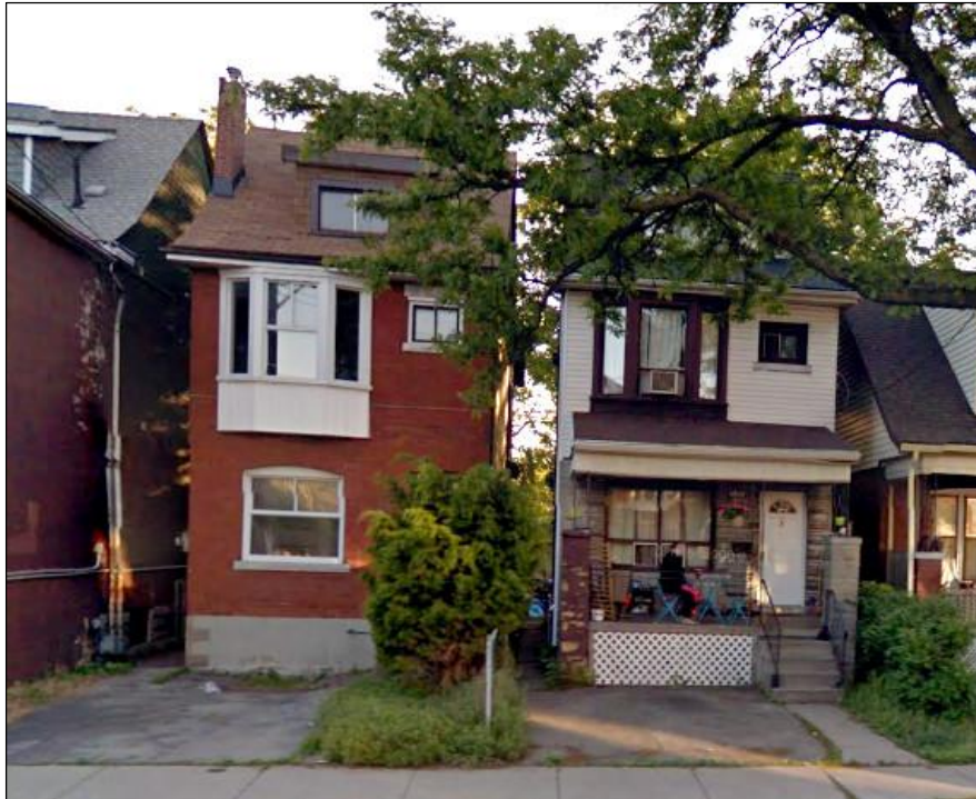
Photograph 3: Façades of 1201 and 1203 King Street East
