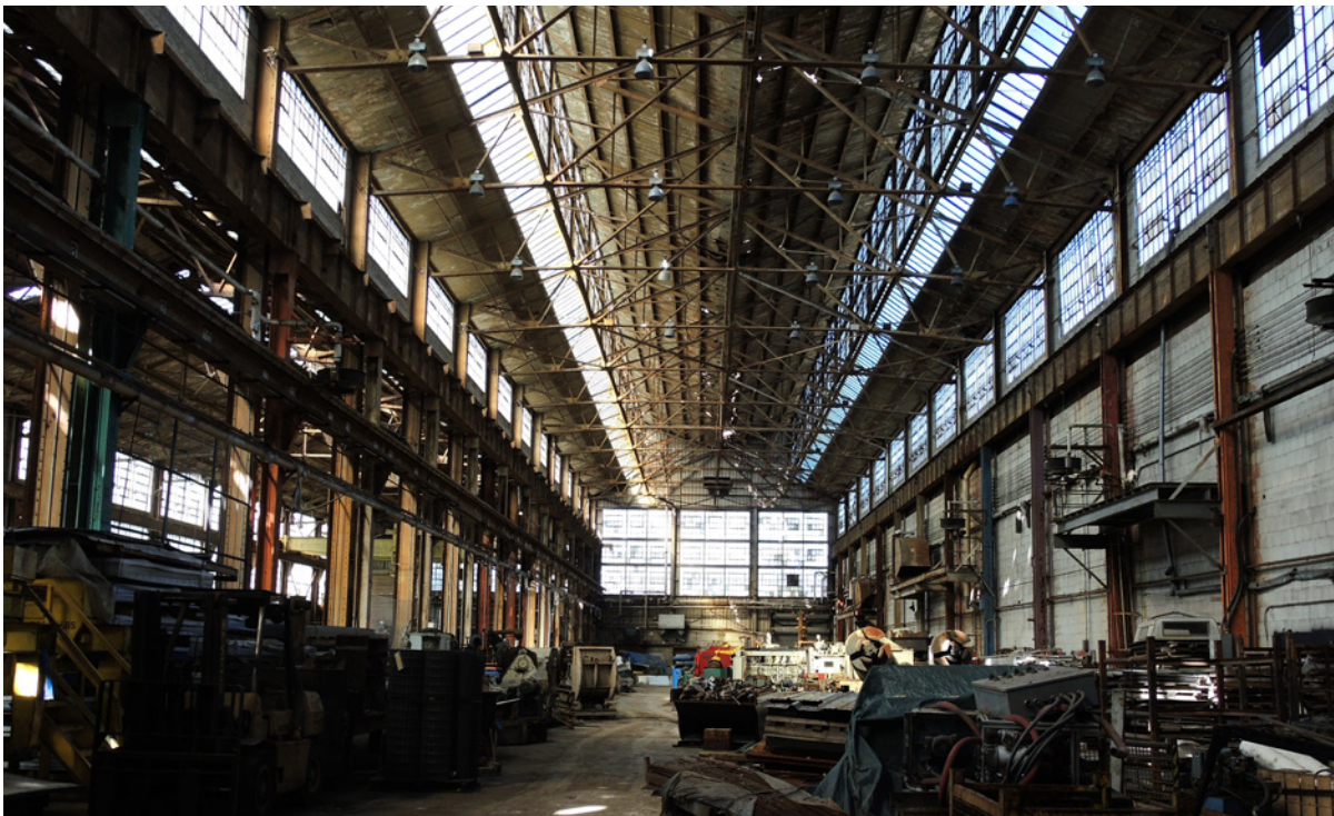
Below: Second production shed, with butterfly monitor roof, looking north, 2016 (ERA Architects)
