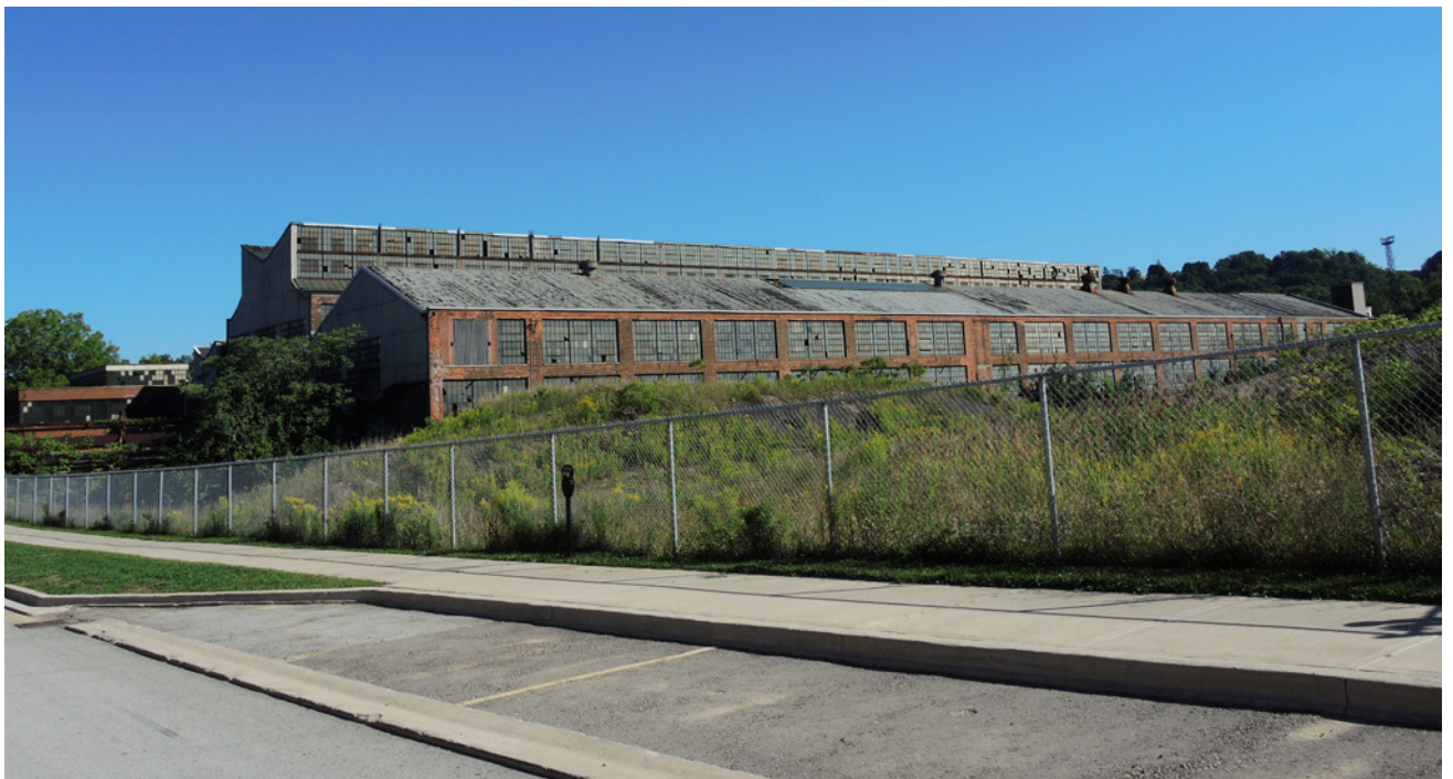
View from the west, 2016 (ERA Architects).
