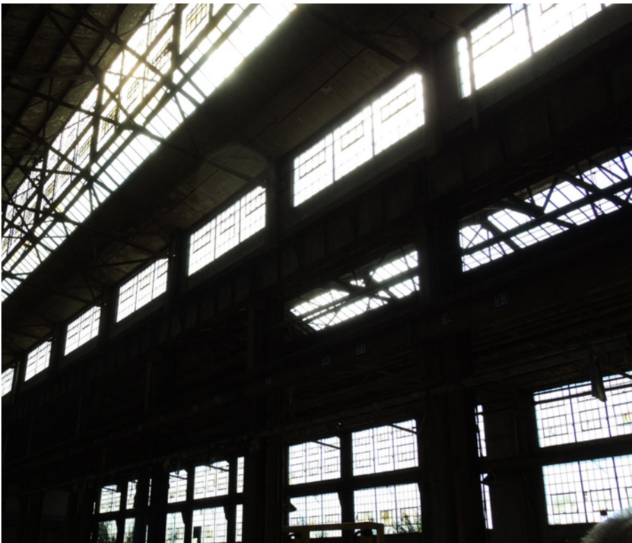
Extensive fenestration systems within production sheds, using butterfly monitor roof system, 2016 (ERA Architects).
