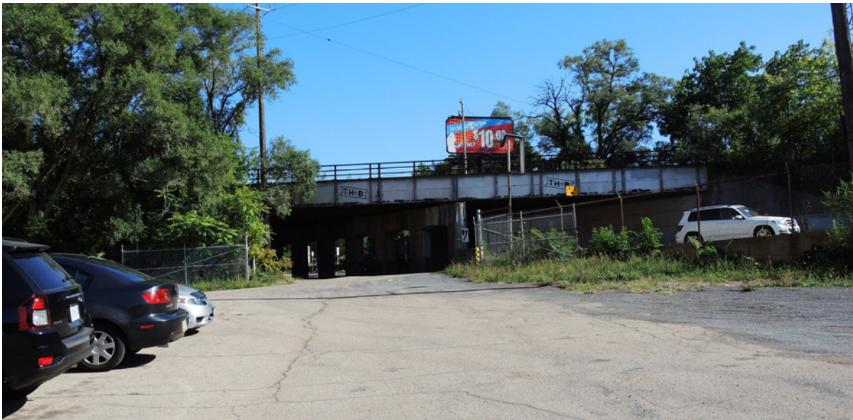
CPR line overpass at Aberdeen Avenue, from the parking lot at 606 Aberdeen Avenue, 2016 (ERA Architects).
