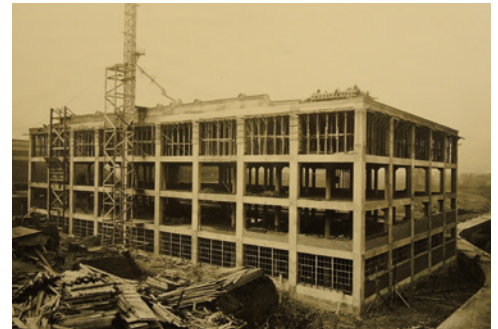
11. West Plant under construction (McMaster Westinghouse archives)
