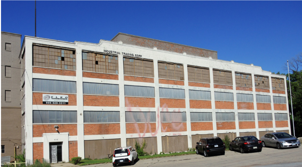
South elevation; looking north east from Aberdeen Avenue, 2016 (ERA Architects).
