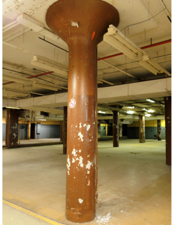
L: West stairwell of Aberdeen frontage showing the structure's painted-over west windows; R: Second storey of Aberdeen frontage showing mushroom column system of the structure's reinforced concrete lofts; Below: ground floor of Aberdeen frontage showing with entrance to rear production sheds, 2016 (ERA Architects).
