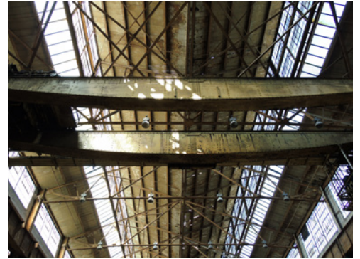
8. Overhead traveling crane in steel-frame production shed with butterfly monitor roof, 2016 (ERA Architects).
