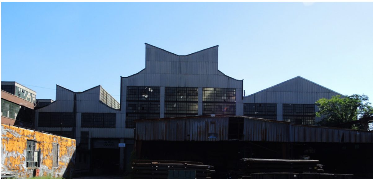
North elevation, showing multiple roof forms of the foundry production sheds, 2016 (ERA Architects).
