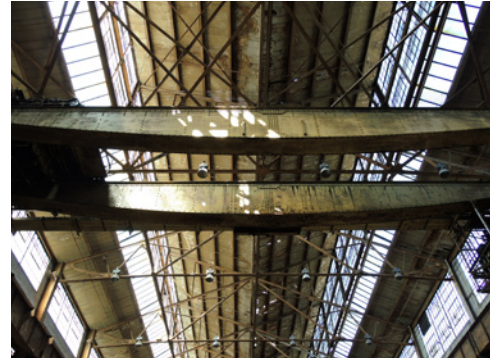
Production shed with butterfly roof, complex fenestration system and traveling crane, 2016 (ERA Architects)
