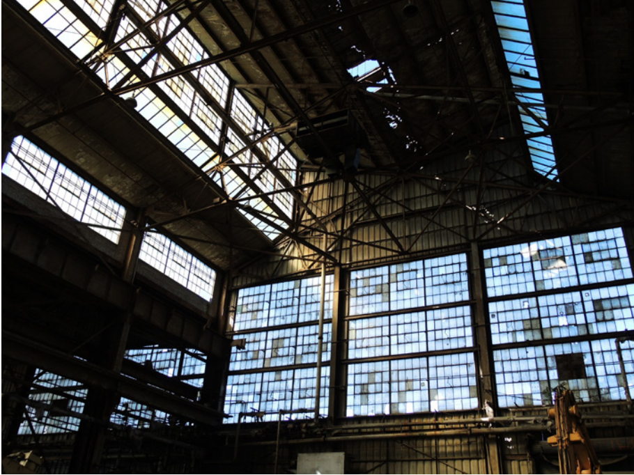
Extensive fenestration systems within production sheds, using butterfly monitor roof system, 2016 (ERA Architects).
