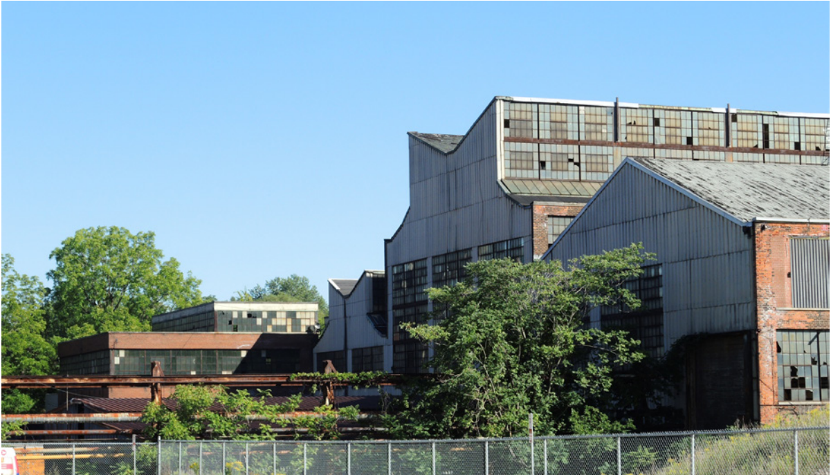
Partial north elevation; looking south east from Frid Street, 2016 (ERA Architects)
