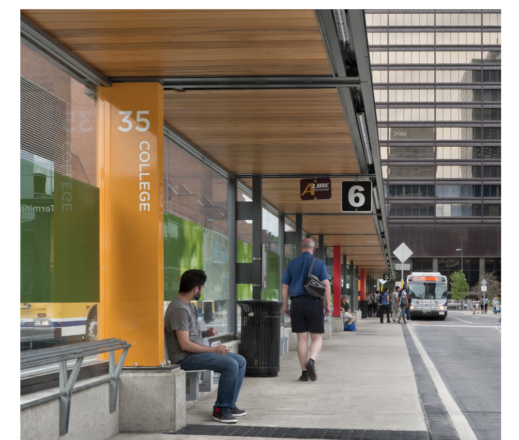
↑ Precedent example of well designed Stops, Hamilton
