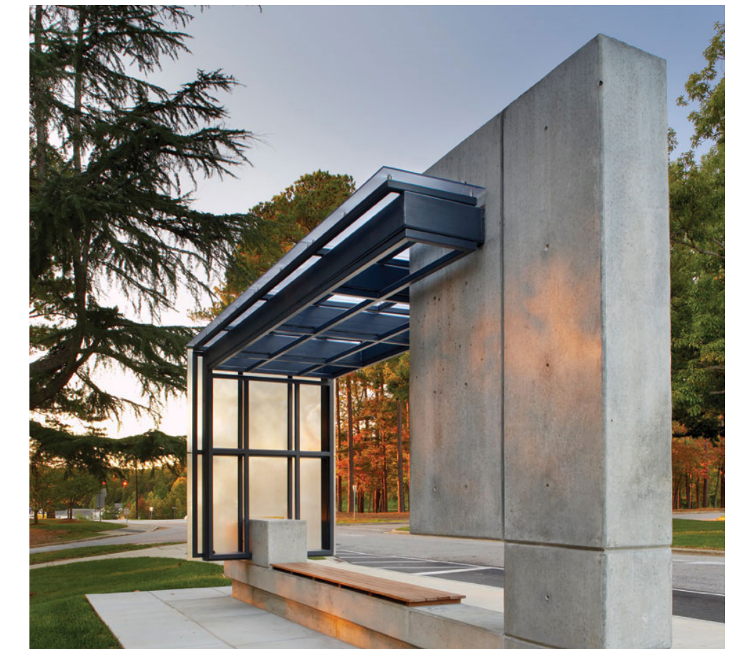
↑ Precedent example of well designed Stops, Raleigh, North Carolina
