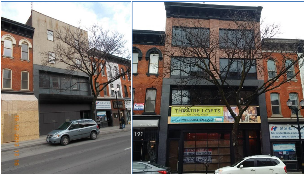
193 King Street East, Hamilton (before and after)
