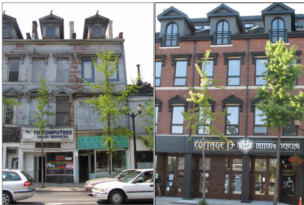
103-107 James Street North, Hamilton (before and after)
