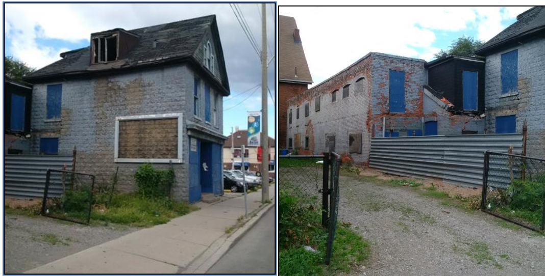
374 Barton Street East, Hamilton (existing conditions)
