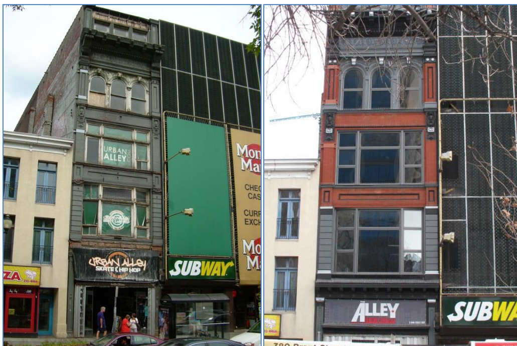
11 King Street East, Hamilton (before and after)
