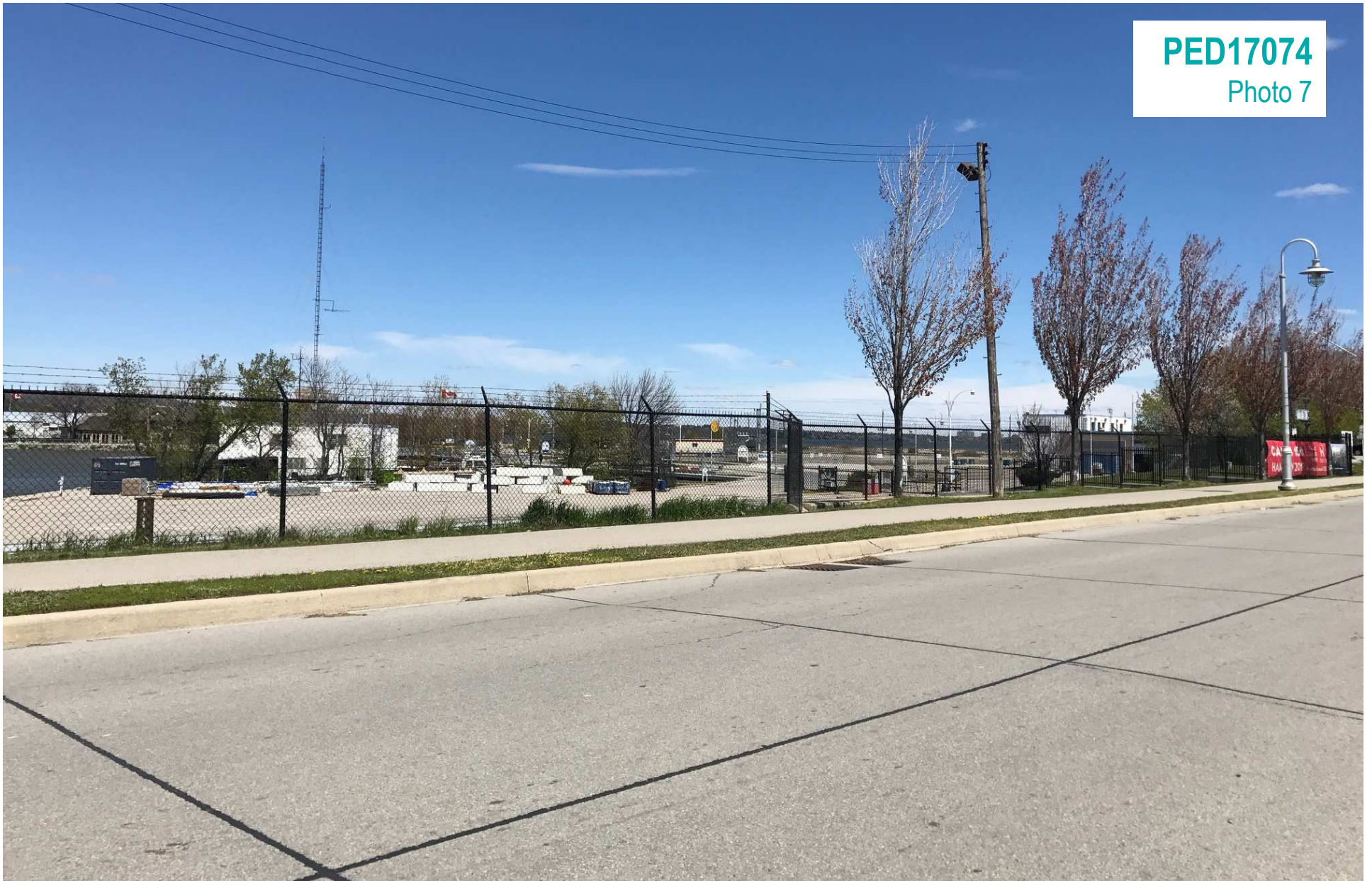
View North Across Pier 7 & 8
