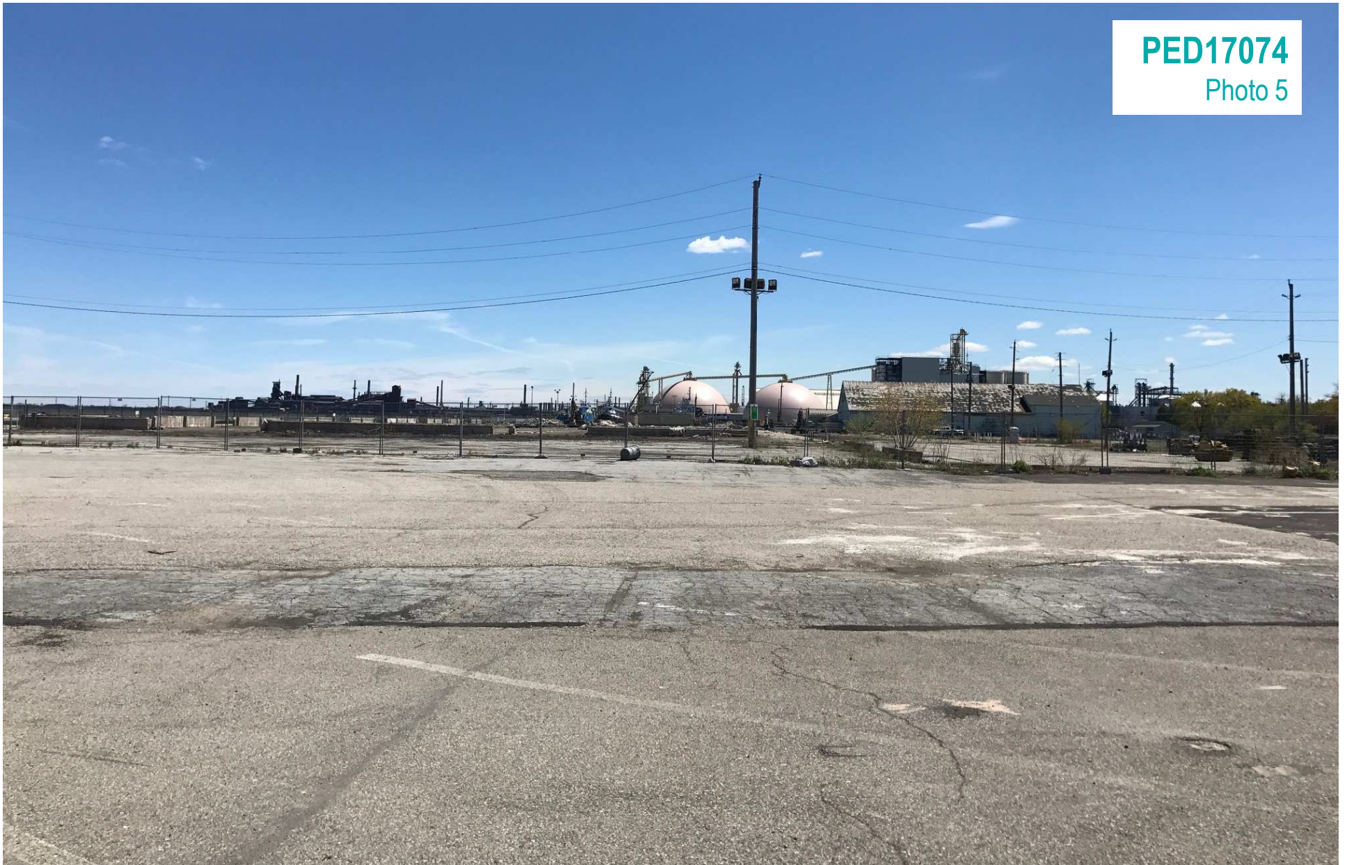
View East towards Pier 10
