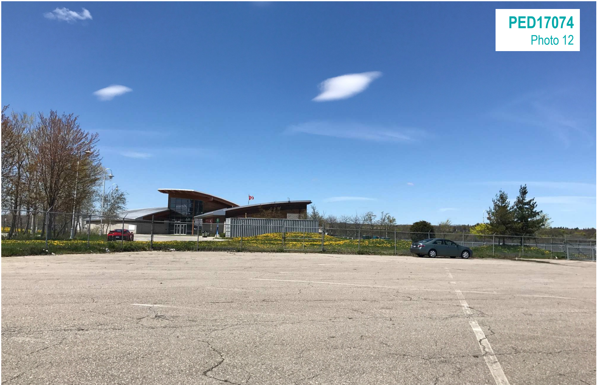
View West across Pier 8
