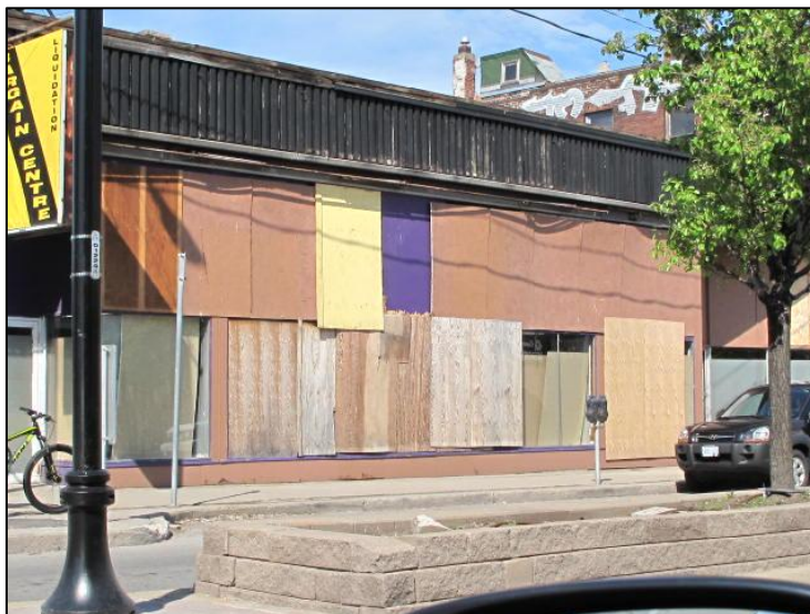
Existing conditions 423-429 Barton Street East, Hamilton
