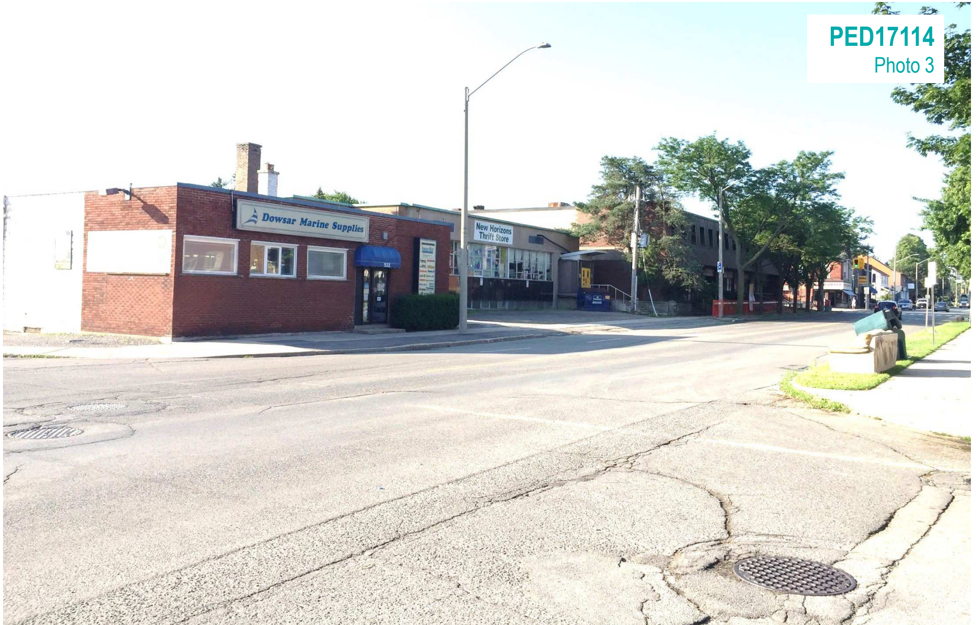
Subject Site – Looking Southeast towards subject site from James Street North and Macaulay Street
