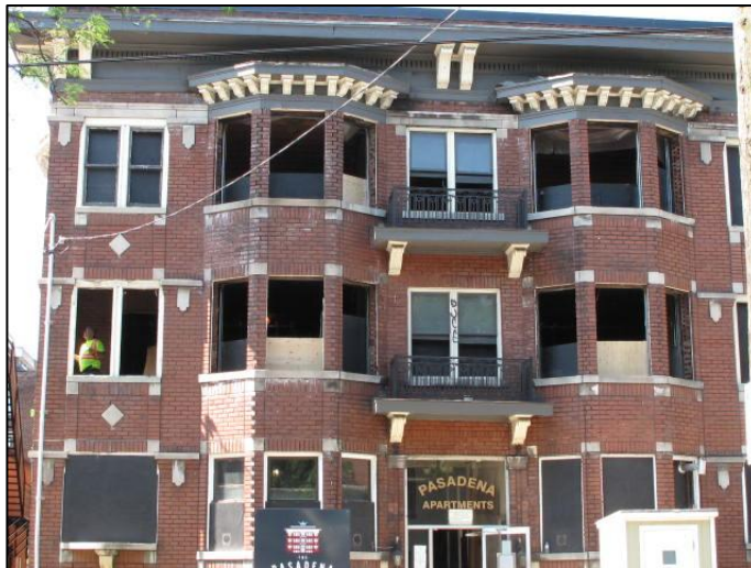
Existing conditions – 27 Bold Street
