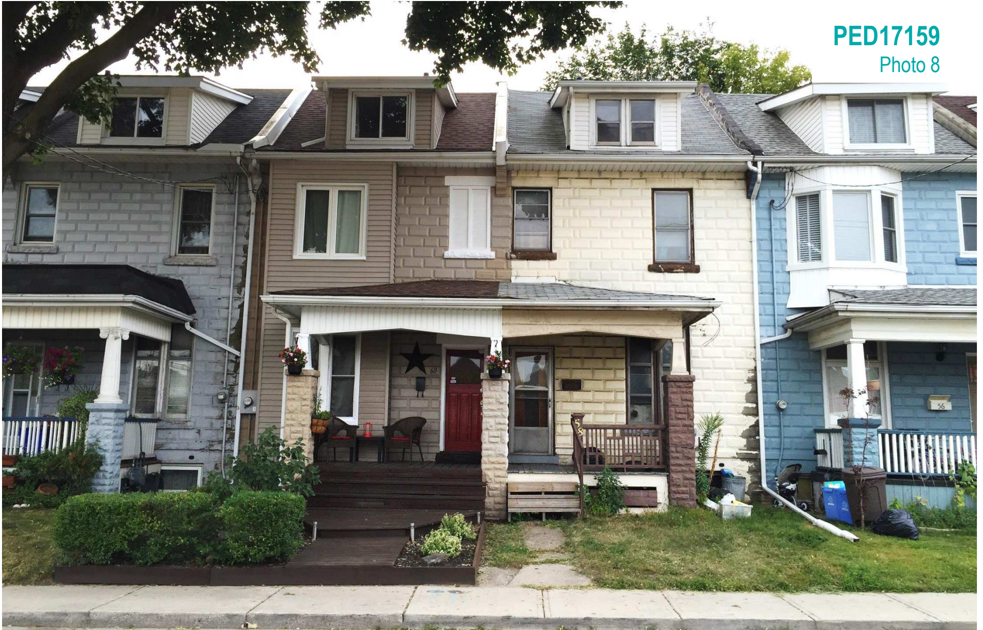
Looking directly at 58 and 60 Gibson Avenue located directly East of subject site
