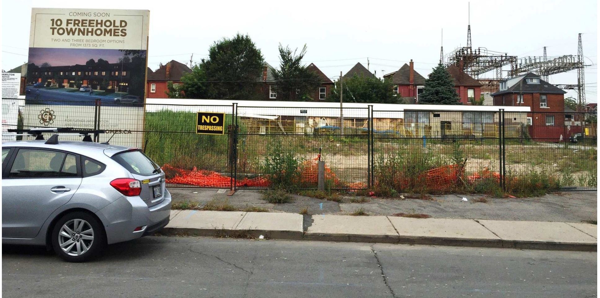
Looking West directly towards subject site from Gibson Avenue
