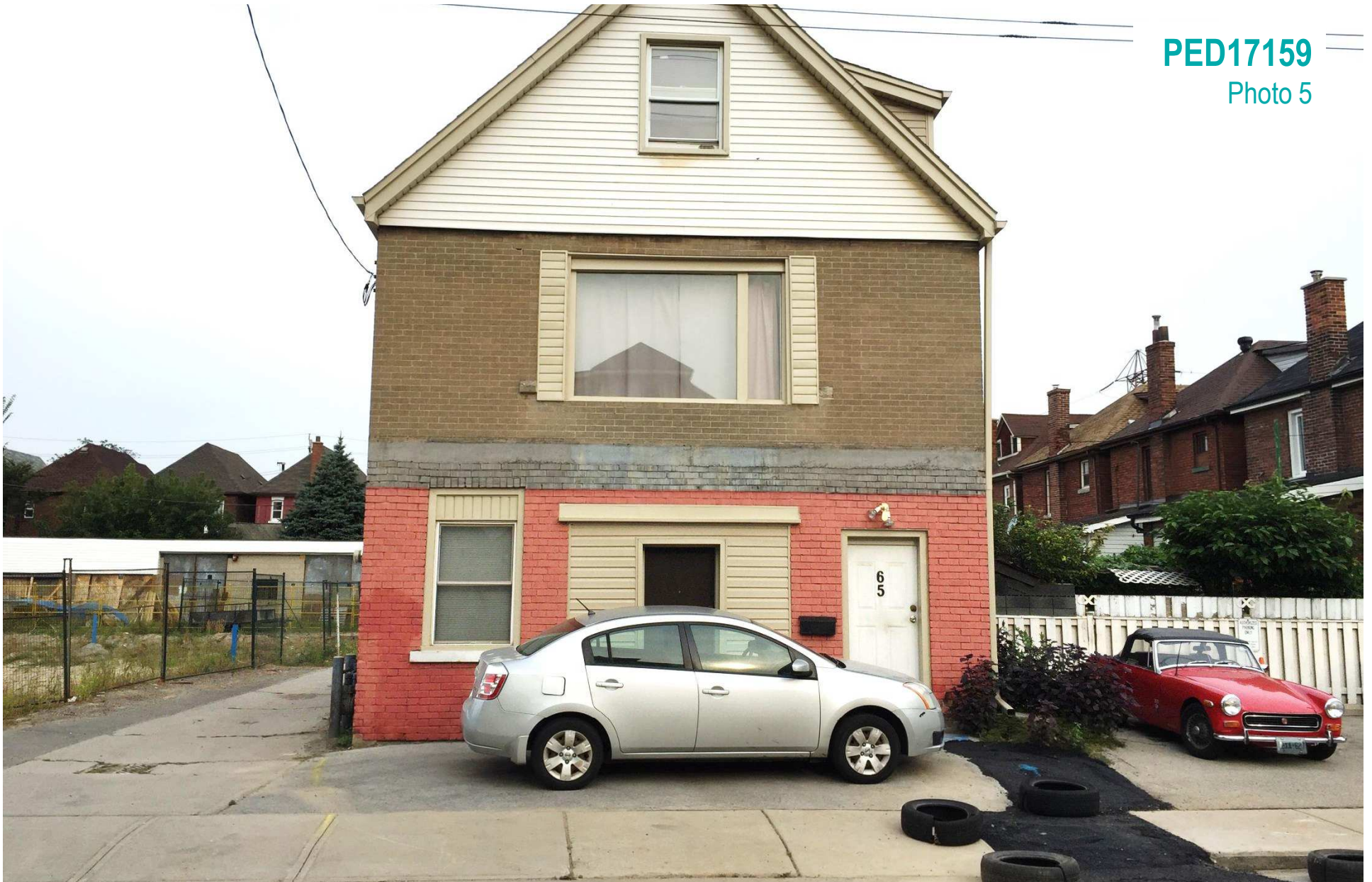
Looking at 65 Gibson Avenue, located North of subject site
