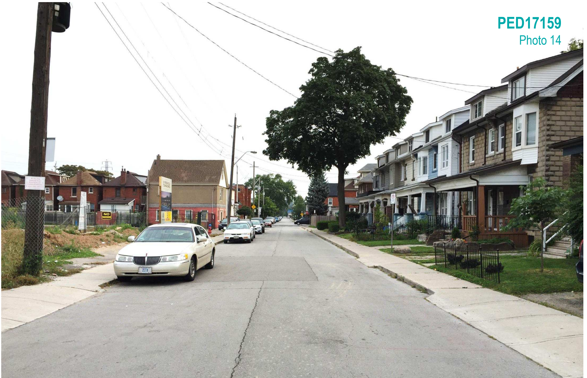
Looking North on Gibson Avenue, subject site is located on the left side
