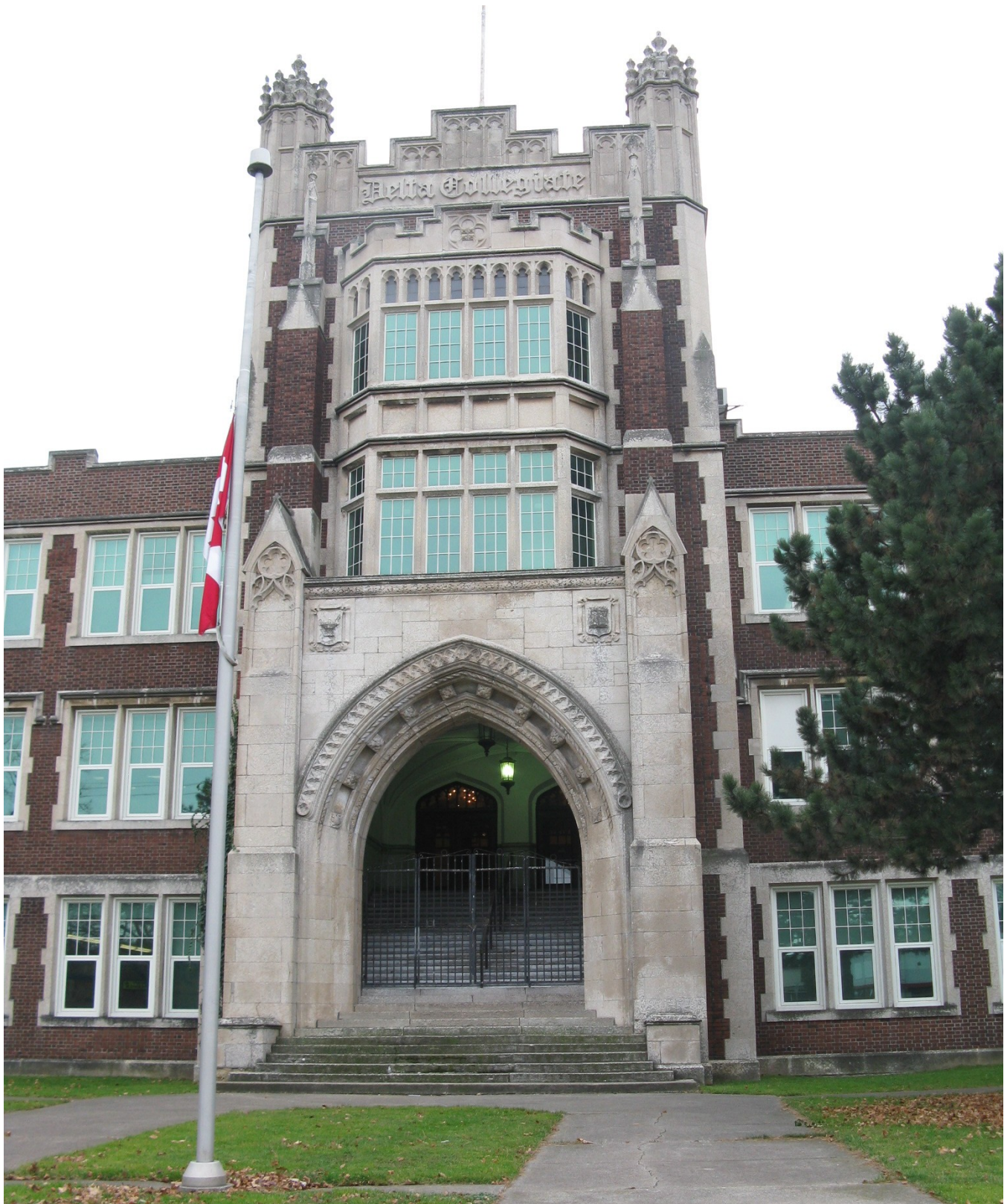
Delta Secondary School – North façade, central entrance onto Main Street East
