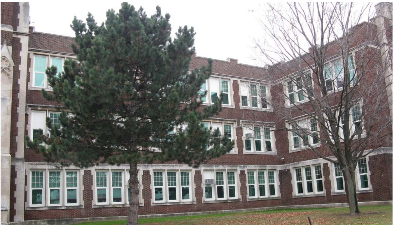
Delta Secondary School – North east façade of 1924 building fronting onto Main Street East
