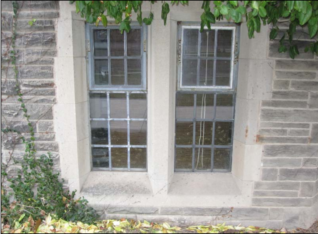
University Hall - detail of the existing windows on the lower level
