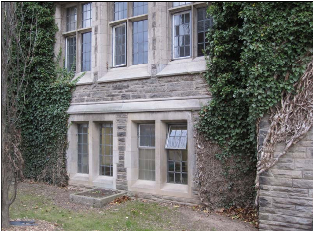
University Hall - detail of the existing windows on the lower levels
