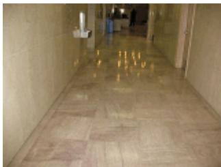
Marble floor covering provided in the corridors.
