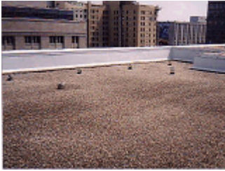
General view of the upper main Built Up Roof.
