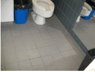
Typical condition of the ceramic floor tiles provided in the washrooms.
