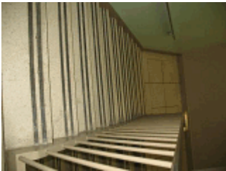
Metal framed stairs with terrazzo treads.
