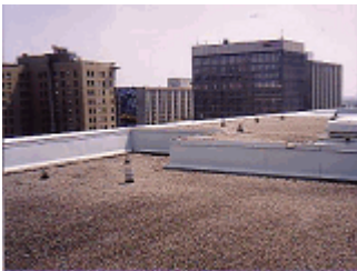
General view of upper penthouse
