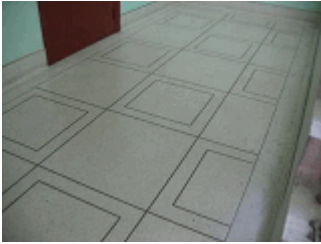
Terrazzo floor covering in the basement.
