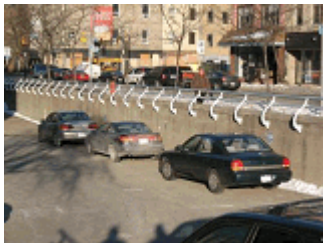
Poured concrete retaining wall provided on the east and west property perimeter.
