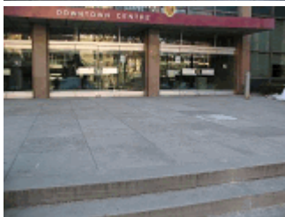
Queenston unit pavers provided at the main building entrance.
