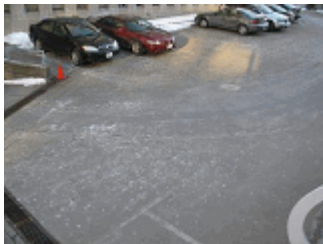
General condition of the asphalt paved parking surface.
