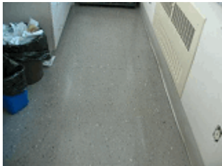
Condition of vinyl floor tile provided in the building.
