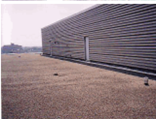
General view of the upper main roof.
