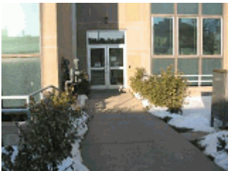
Aluminum door with IGUs on the south elevation.
