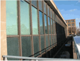
Typical window wall system seen on the south elevation.
