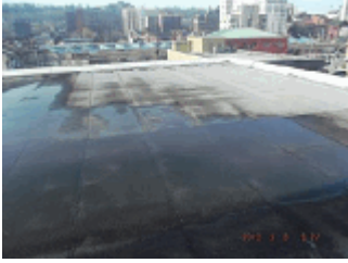
Portion of level 2 roof appears to have been replaced.
