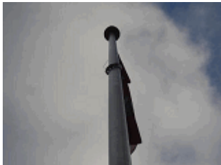
Photo 11 - top of pole
