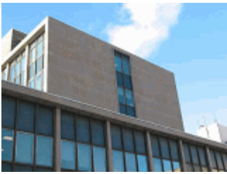
Granite stone facing provided on the exterior walls on all elevations.
