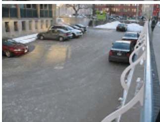
General condition of the asphalt paved concrete surface.
