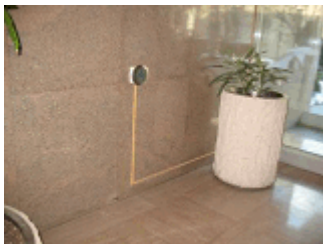
Portion of the marble floor covering seen in main entrance foyer.
