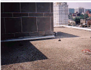
General view of the upper main roof.
