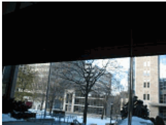
Air leakages experienced at door interfaces.
