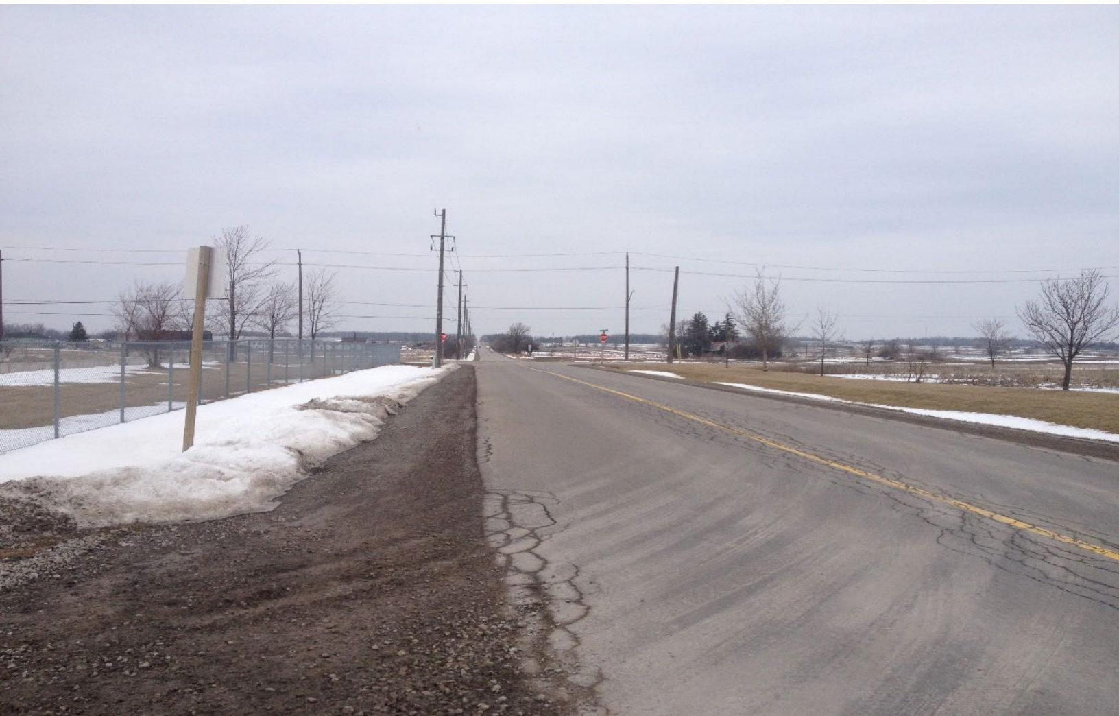
Figure 30: First Road East - Looking North
