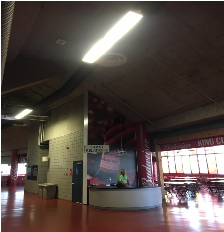
Photo: Level Three Concourse Stairwell beside Existing Passenger Elevator Proposed Location of New Passenger/ Service Elevator(s) to Service Levels 1-4
