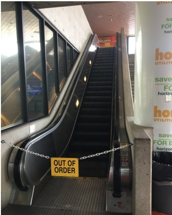
Escalator #4 – Bay Street South
