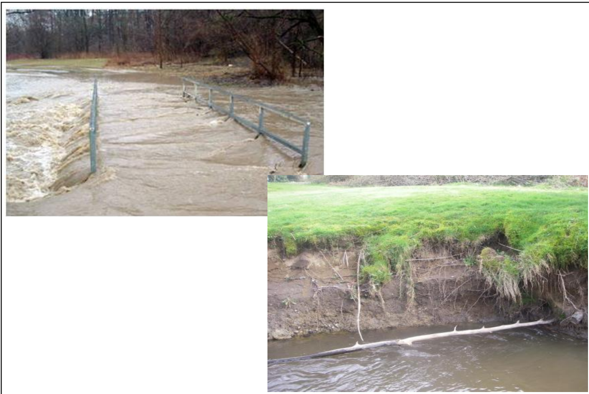
Figure 5.3: Flooding and Erosion Impacts
