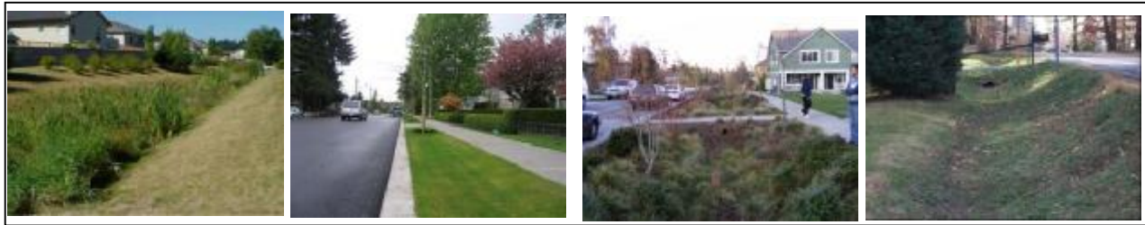
Figure 6.4: Example LID Conveyance Controls (From L to R: Vegetated Channel, Subsurface Perforated Pipe, Bio-swale, Grass Channel)
