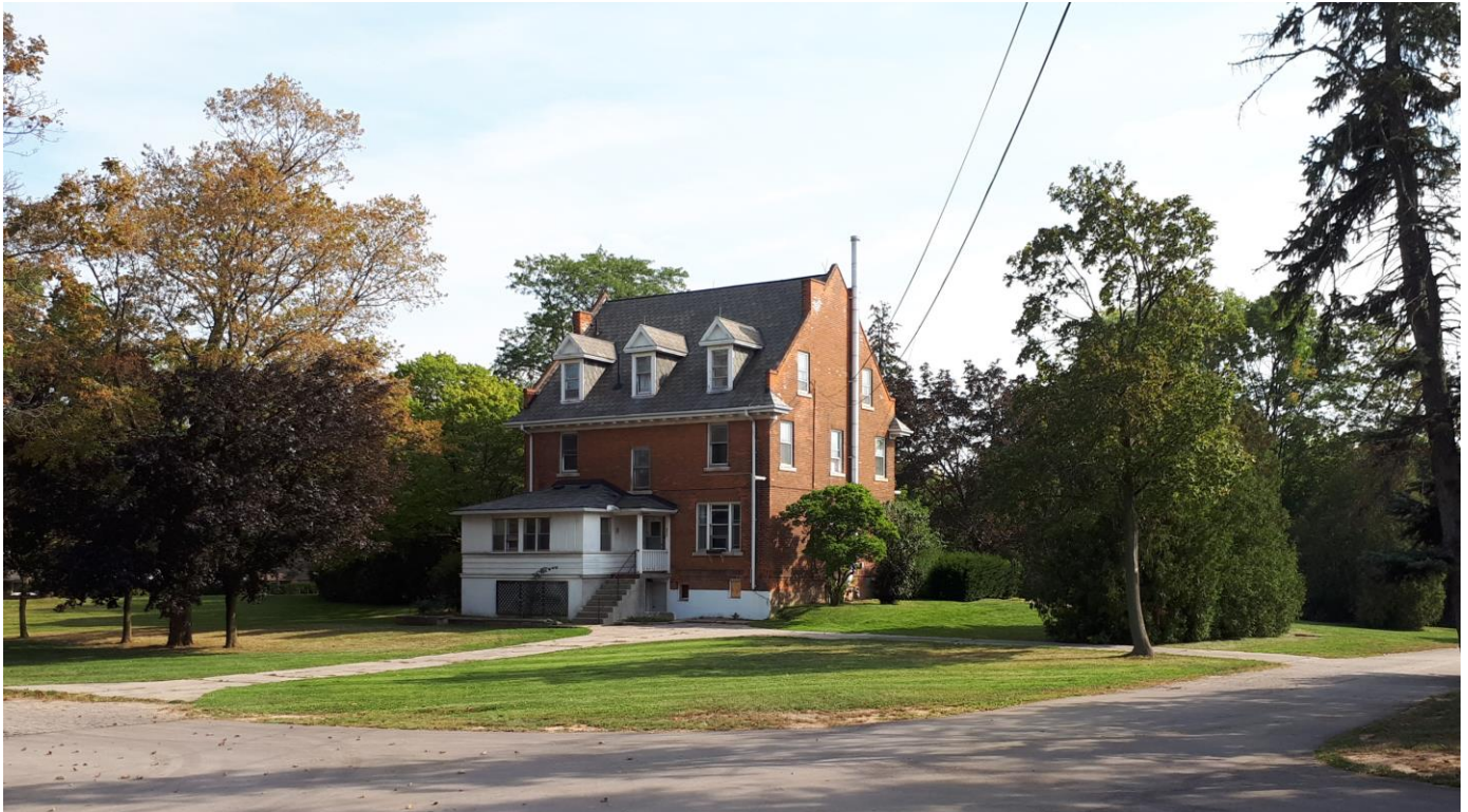
Figure 4: View of the rear of the building (north and west elevations) showing a matching profile with equivalent pedimented dormers. An early one-and-a-half storey aluminum and wooden-clad addition is shown on the eastern portion of the rear façade (2017).
