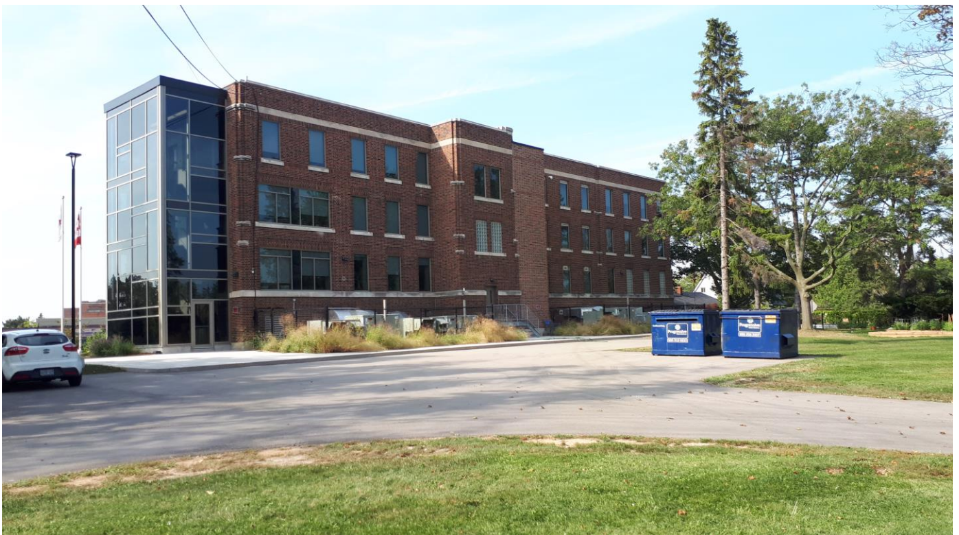
Figure 15: The rear (east) portion of the building. Note the modern addition, off-colour brick elevator addition, and modern windows. The brick building features a simple rear façade with stone sills, soldier course brick lintels, and stone stringcourses running the length of the façade (2017).
