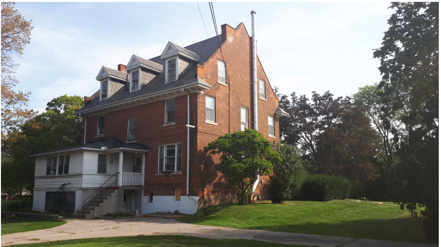
Figure 5: A closer look at the rear of the building (2017).
