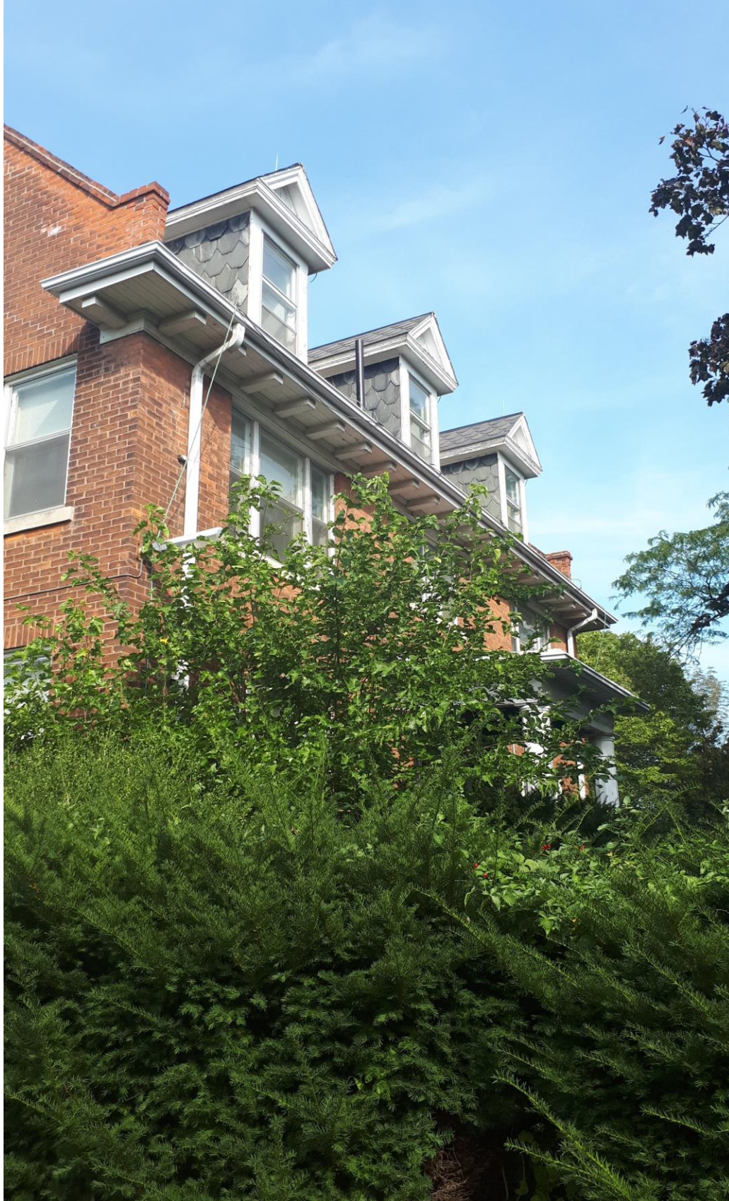
Figure 3: View from the southwest corner of the roofline profile. The image displays slate siding on the dormers, projected brick corbel corners, and modillion brackets on the underside of an extended cornice soffit (2017).
