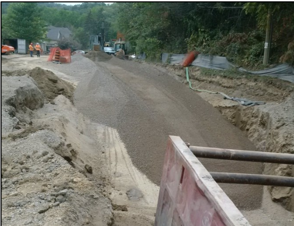
Montgomery Drive Reconstruction
