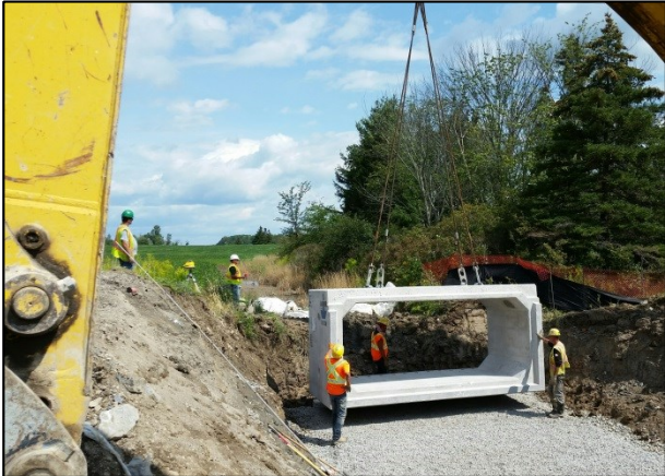
Bell Road Culvert Replacement
