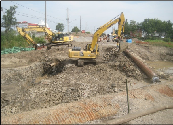
Dartnall Road Culvert
