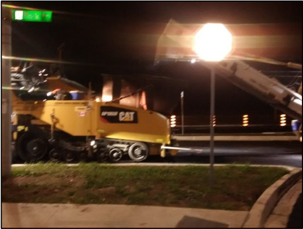
York Boulevard Reconstruction
