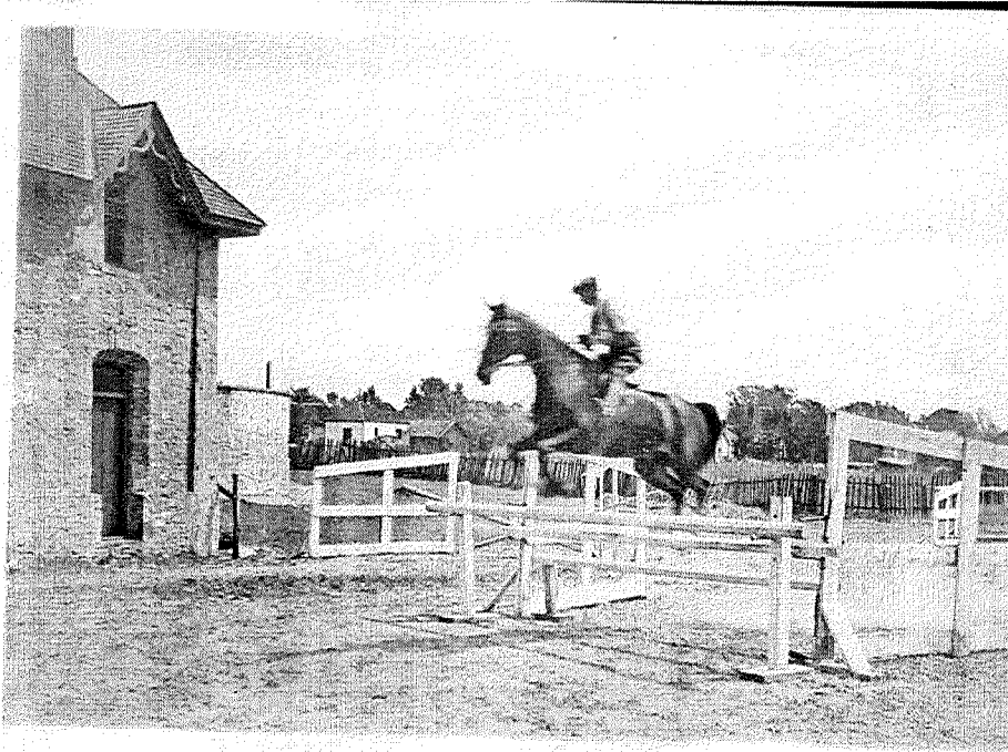
Dovecote in its original condition at left hand side of photograph.
