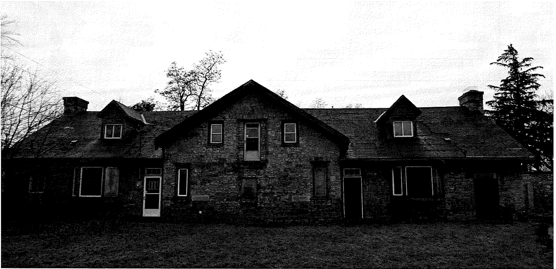
East elevation - Repair of roof required, block up new openings and restore original openings, repoint 25% of exterior stone.
