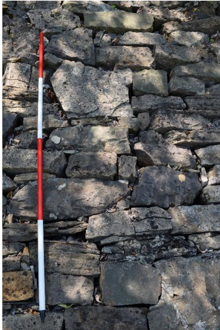
*Figure 27: Detail of the coursed rubble construction.*
