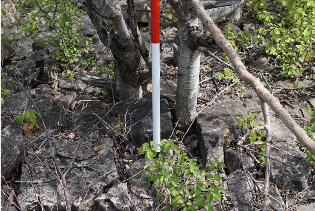
*Figure 71: Root action dislodging stones of the coursed rubble lining of Barton Reservoir.*
