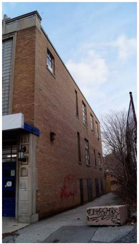
Fig. 75 South or rear elevation of 1951 wing. Note how the front doorway's stone embrasure wraps around the corner to the south elevation and how the stone cornice also does the same.
