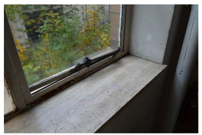
Fig. 135 Detail of window in ground-floor lobby. Note bronze hardware for the operable sash as well as the travertine marble sill.
