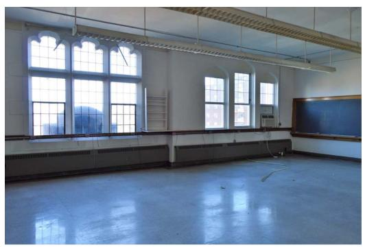
Fig. 110 Room 28 tripartite windows. Note that the sash on the left is original and the sash on the right is a replacement.
