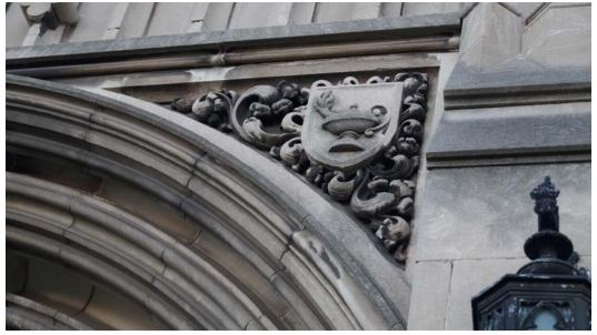
Fig. 31 Triangular stone panel (spandrel) shouldering portal's pointed arch and carved with the "lamp of learning" and foliage
