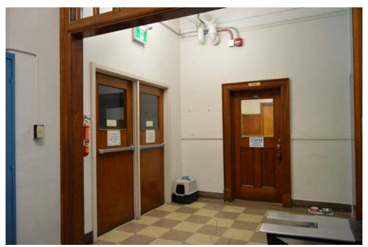
Fig. 79 Place on ground floor where the east-west corridor meets the north-south corridor. Note fire separation partition and fire doors to the left of the frame, door to the administration office, wood-framed transom light over the north-south corridor opening, and terrazzo floor in a checkerboard pattern.
