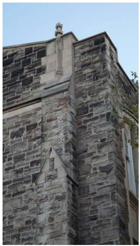
Fig. 49 Gablet on buttress and cap of buttress
