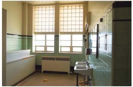
Fig. 147 Upper-floor washroom. Note the green-and-black tiled wainscotting and the window pair with glass block uppers and clear glass lowers.
