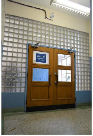
Fig. 132 Ground-floor entrance wall of glass blocks centred by double wood-and-glazed doors
