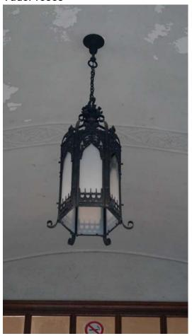
Fig. 38 Entry's porch lamp hanging from vaulted ceiling. Note how pointed arches have been incorporated into the cast-iron lamp.
