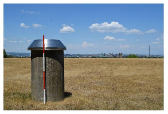
Figure 61: The concrete vent pipes on the north and south boundaries of the reservoir.
