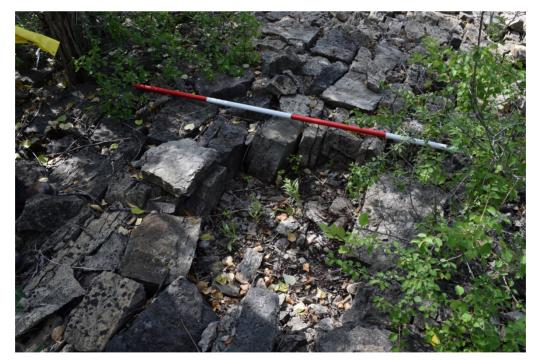
Figure 29: Exposed section of the stone chipping sub-base.
