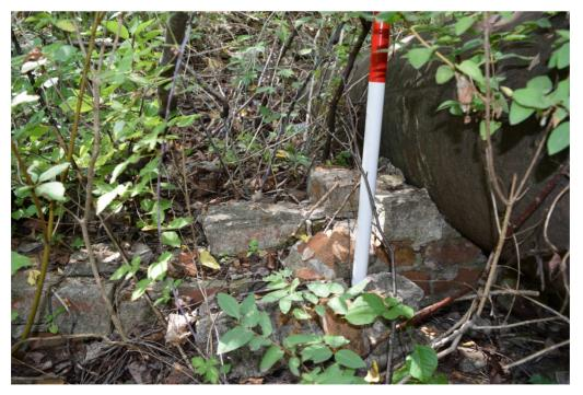
Figure 33: Brick base of the west main pipe.
