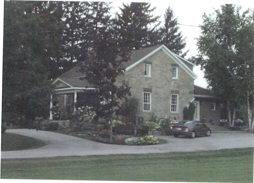
5. Facing southeast corner
