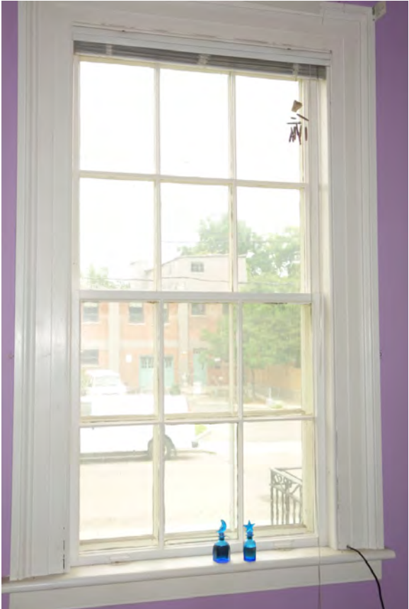
West parlour – 6 over 6 wood sash window
