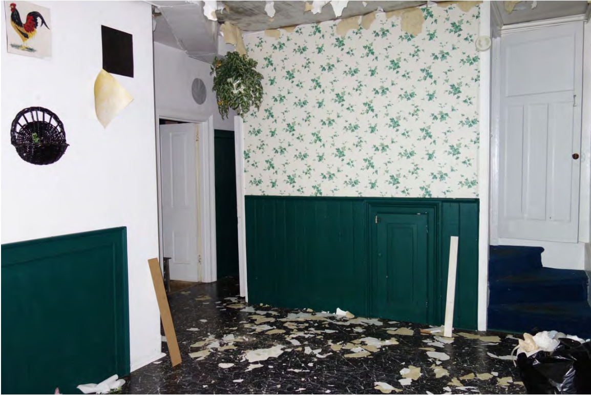
Kitchen – stairs to main floor visible on the right
