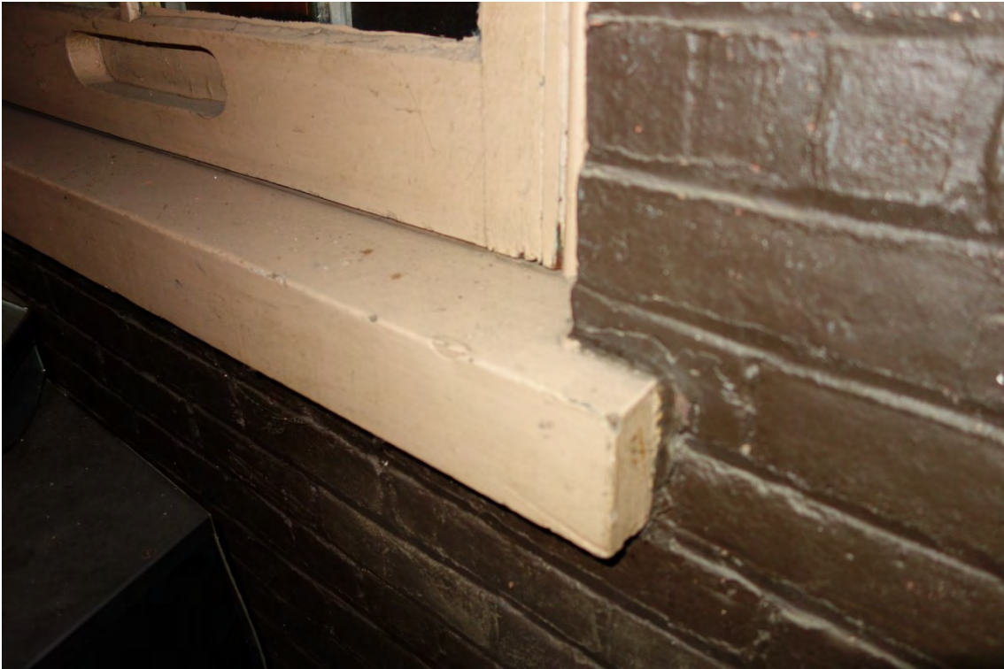
Exterior brick wall - wood window sill
