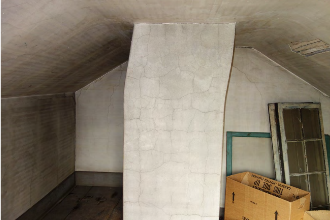
Free-standing chimney stack
