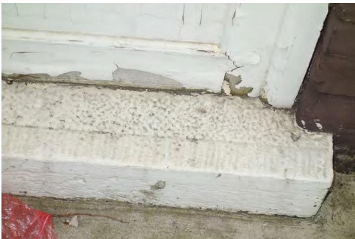
Dressed stone door sill at main entrance
