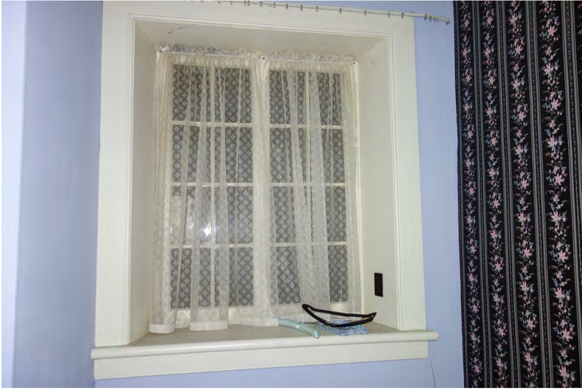
Bedroom 3 – detail of window 2
