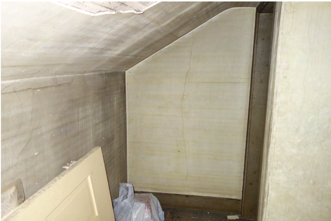
Attic hallway – east end
