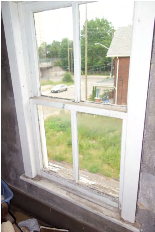
Window – 2 over 2 sash
