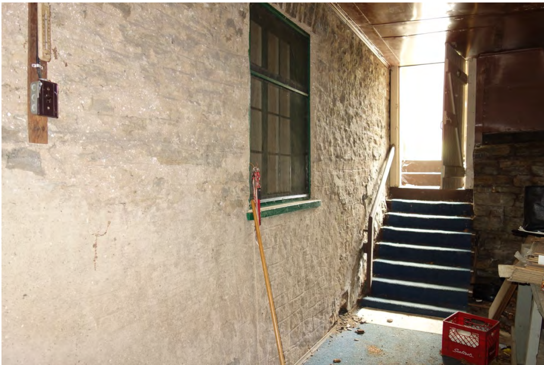
Exterior wall of house - parged rubble stone
