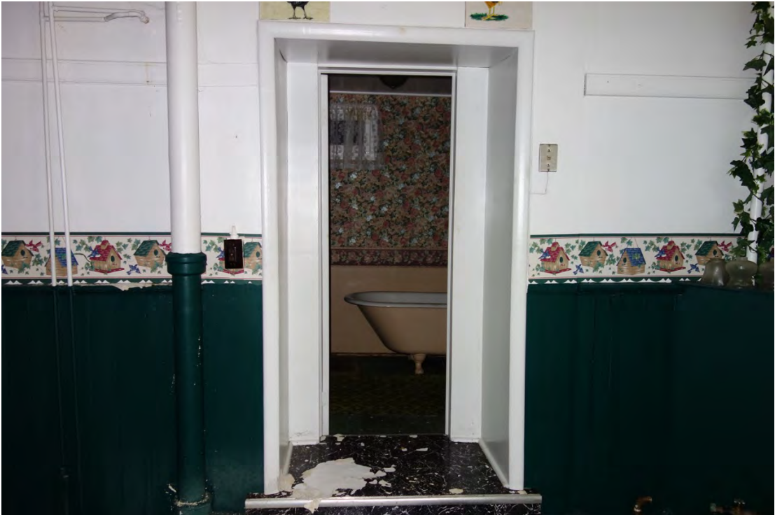
Kitchen – entrance to bathroom that is located in the west end of the porch
