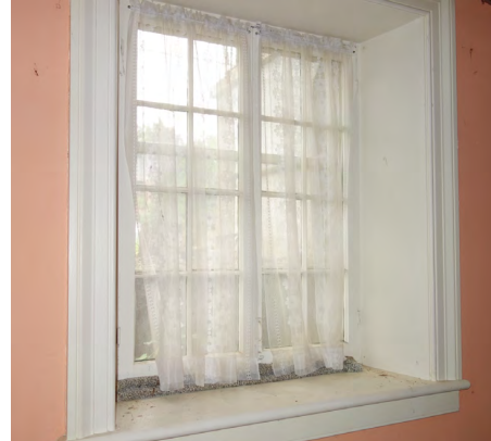
Basement – 8-pane double-casement windows
