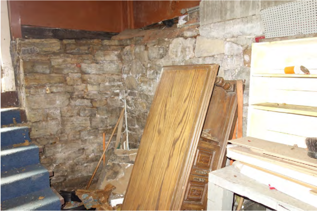
Exterior wall of porch - rubble stone
