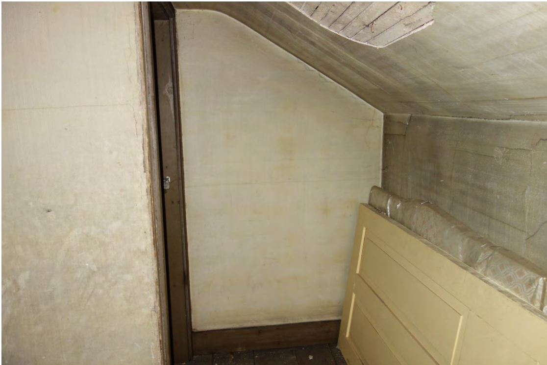
Attic hallway – west end
