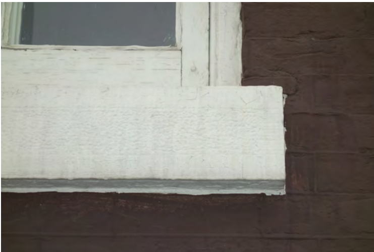
Dressed stone window sill on main elevation
