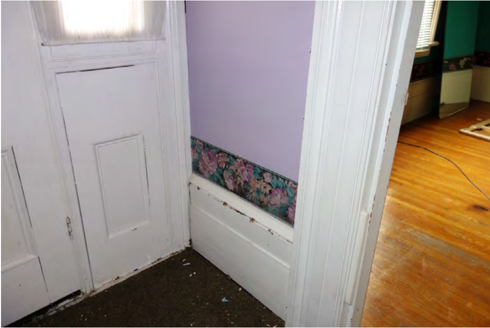
Woodwork in the hallway on the main floor
