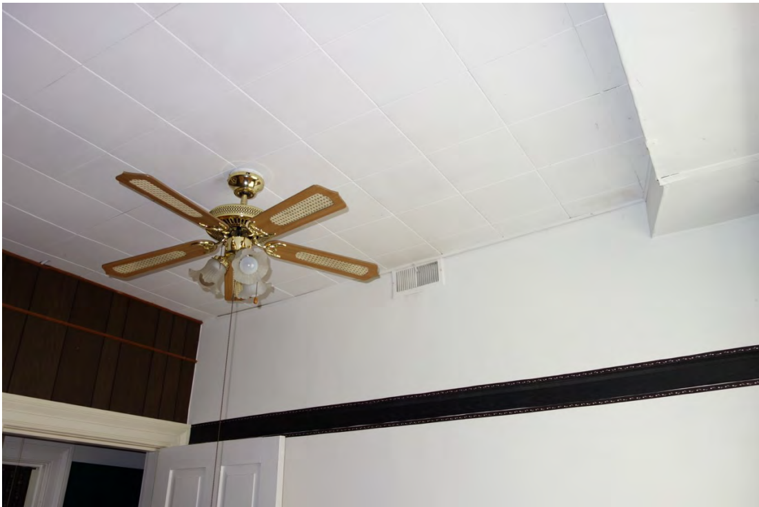
Bedroom 2 – modern ceiling tiles
