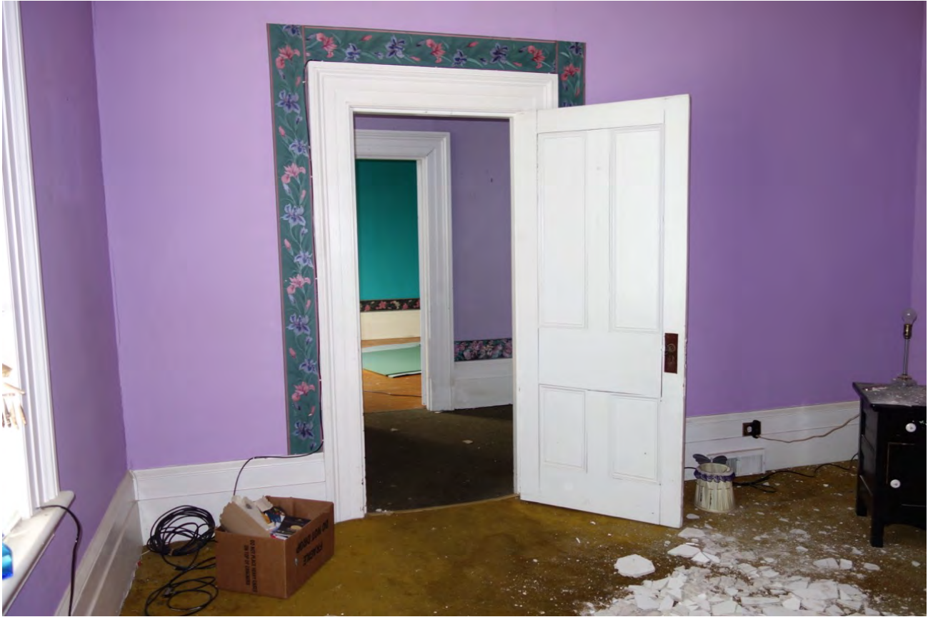
West parlour – door to hallway
