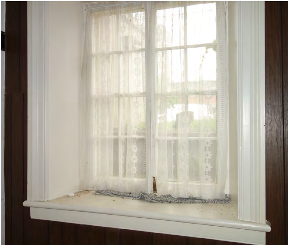
Bedroom 2 – wood casement window
