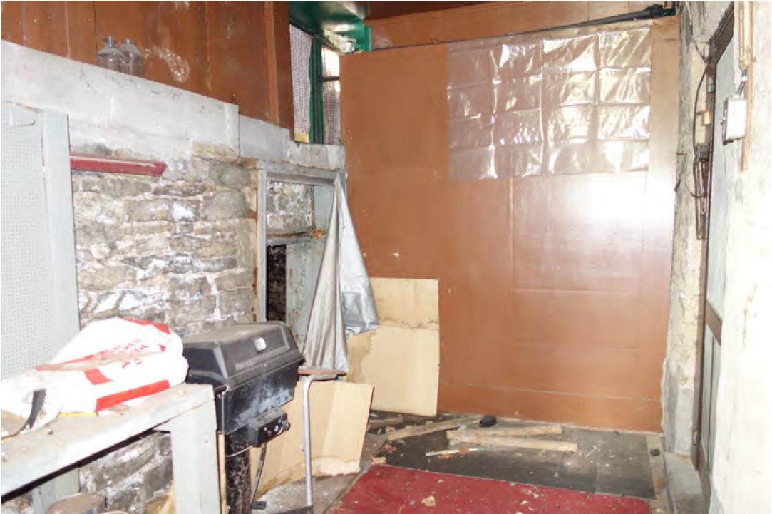
Porch - west end
