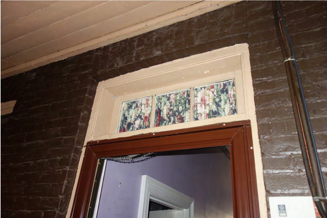
Exterior brick wall visible inside porch – divided transom above the door
