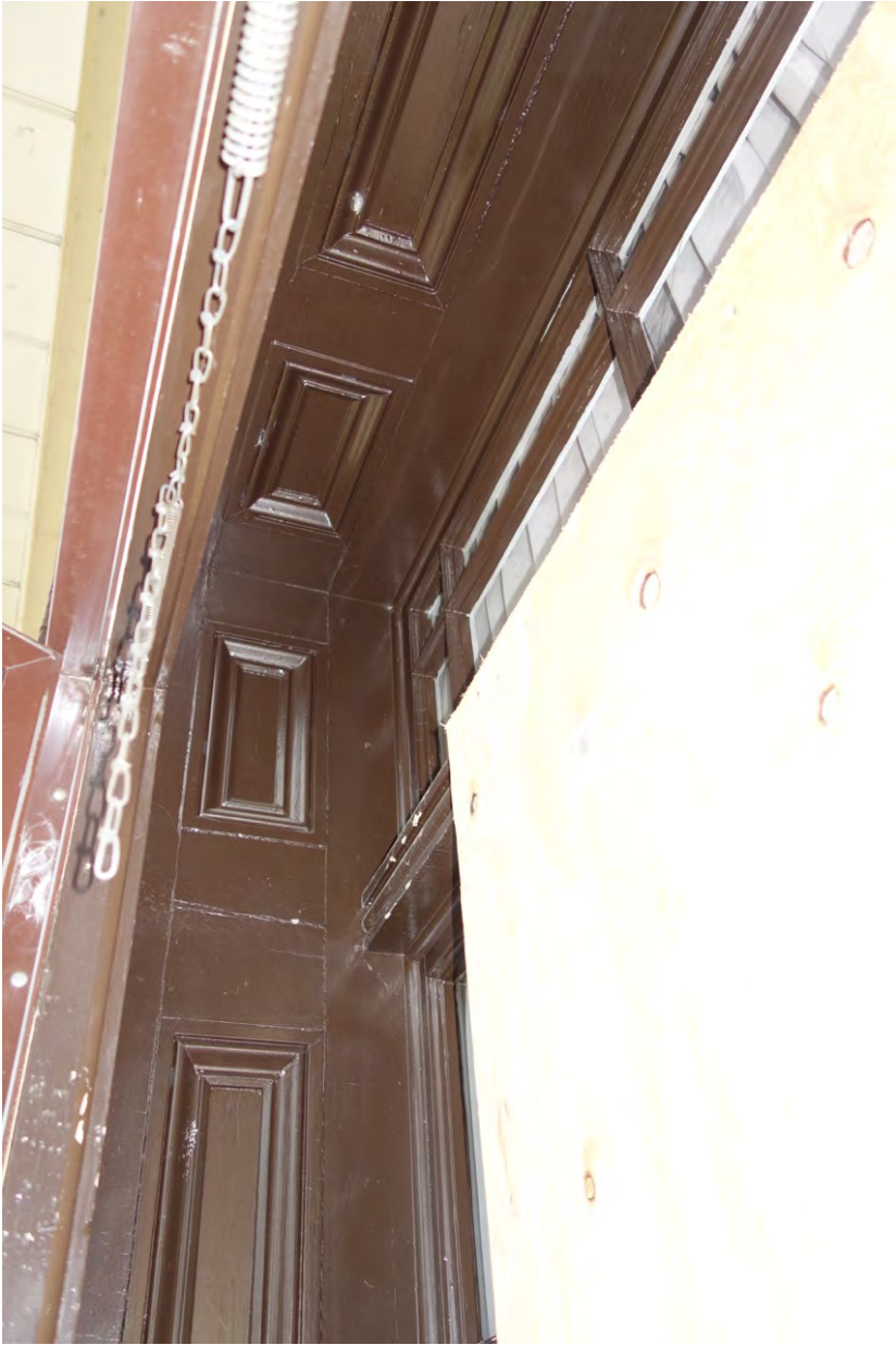
Front entrance wood paneling
