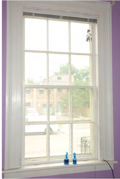
Main floor - 6 over 6 sash windows
