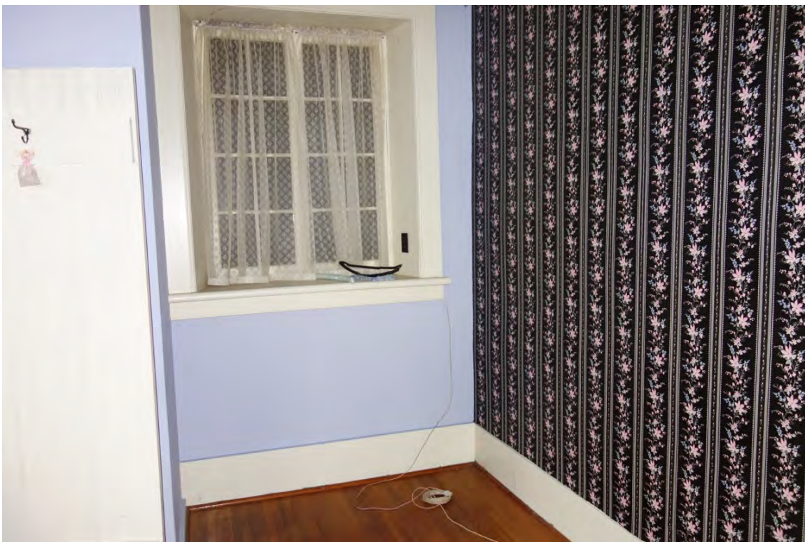
Bedroom 3 – wood casement window 2
