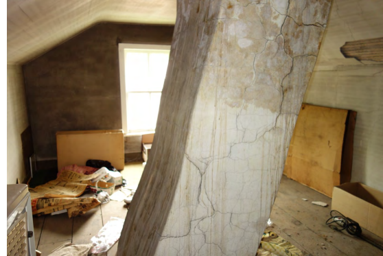
Attic room (freestanding chimney flue)
