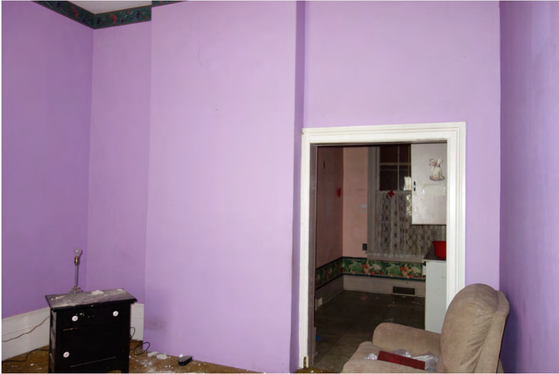
West parlour – dry-wall partition wall containing a chimney
