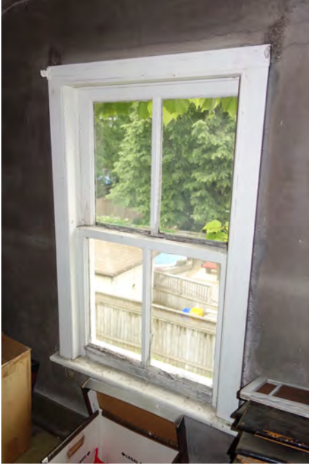
Window - 2 over 2 wood sash
