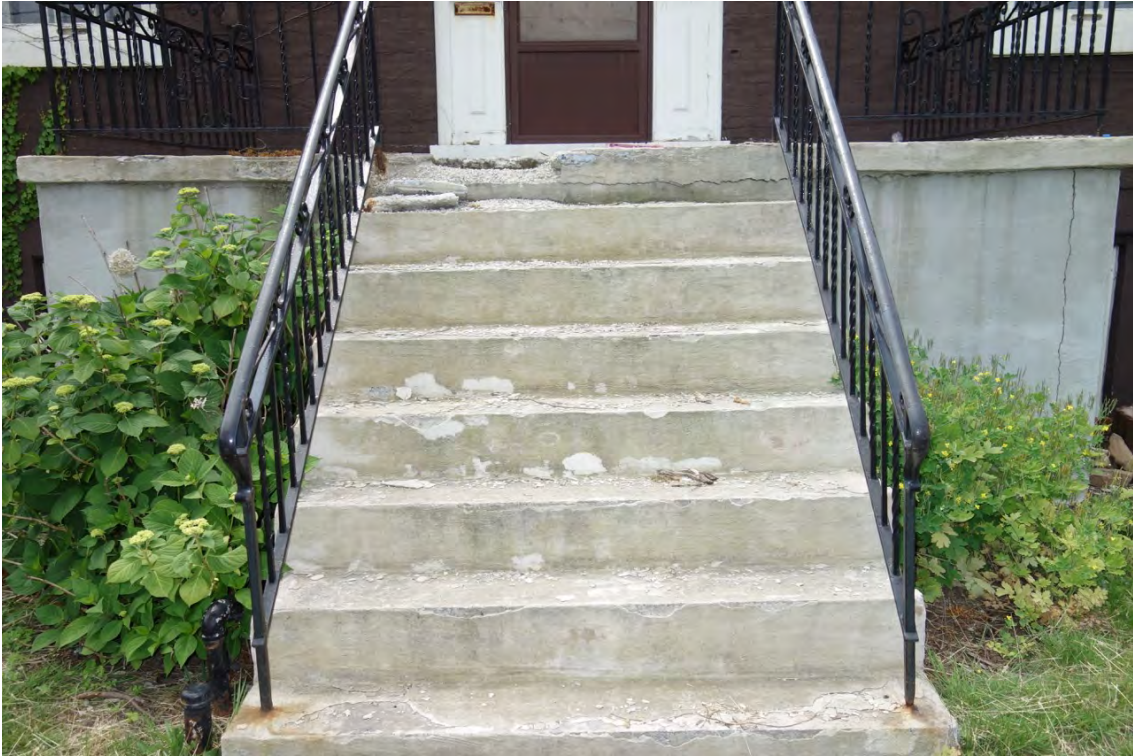
Modern concrete stoop and wrought iron railings
