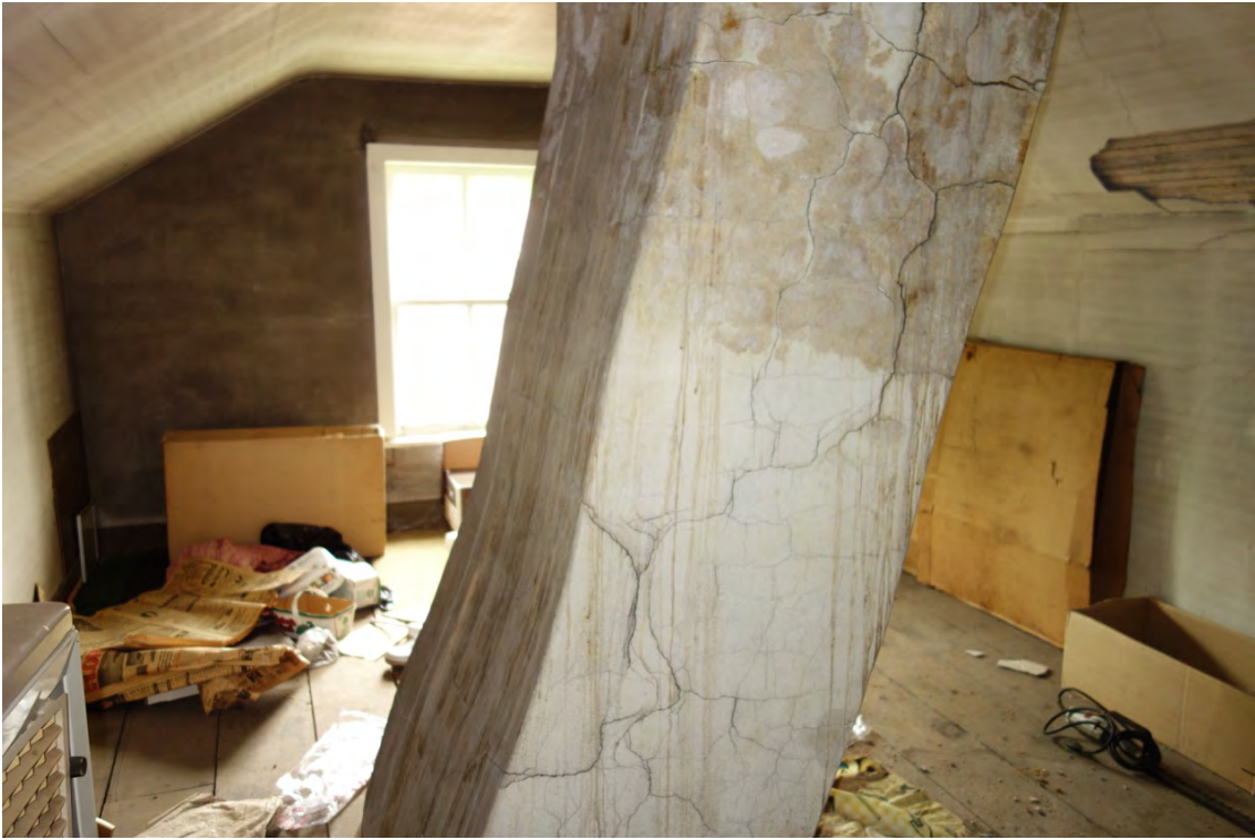
Freestanding chimney stack
