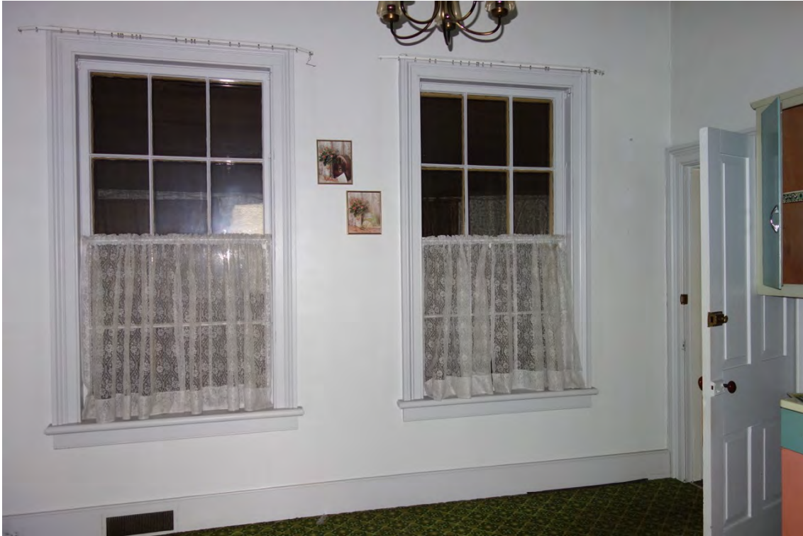
Kitchen 3 – located behind the east parlour – 6 over 6 wood sash windows
