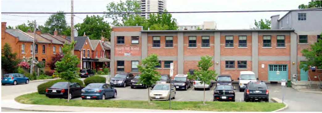
Former Ogilvie Five Roses building, 121 Augusta Street
