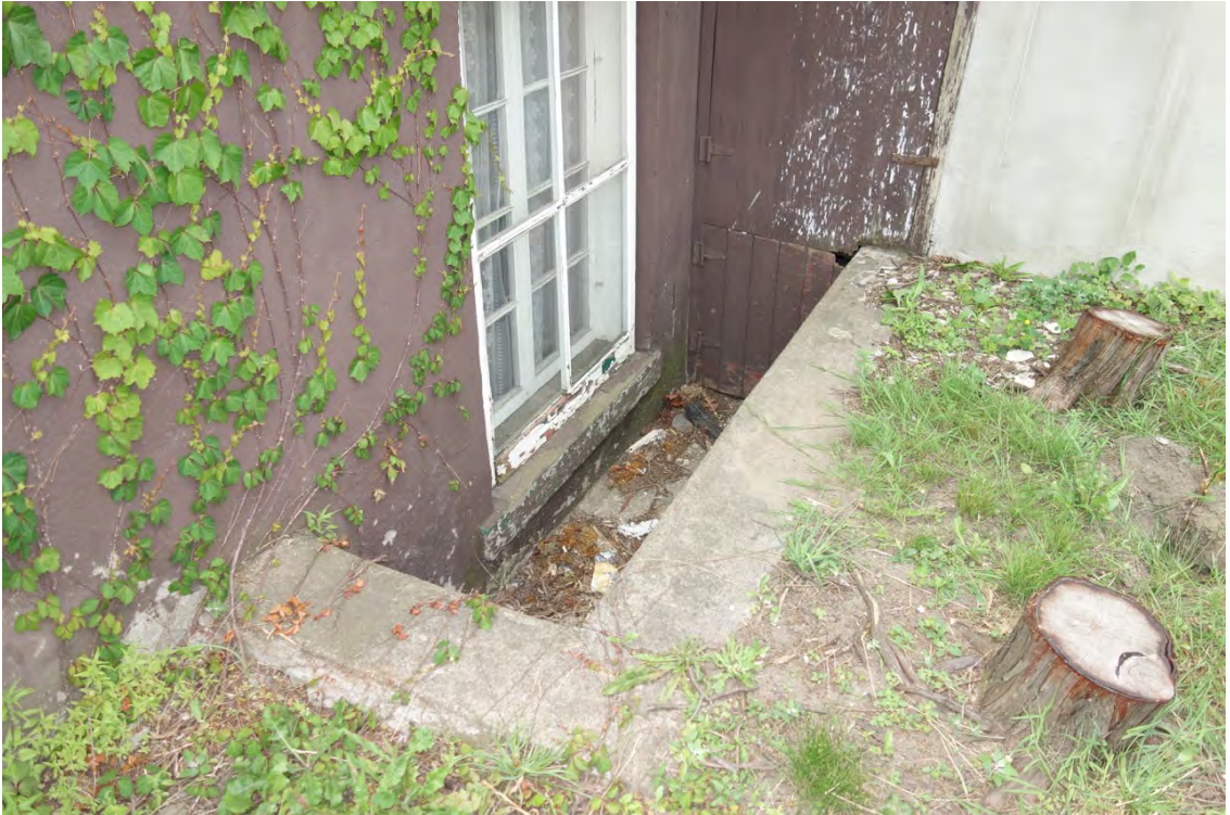
Modern concrete window well
