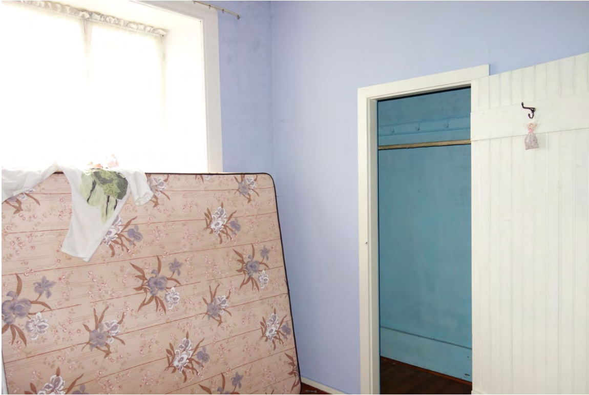
Bedroom 3 – wood casement window 1
