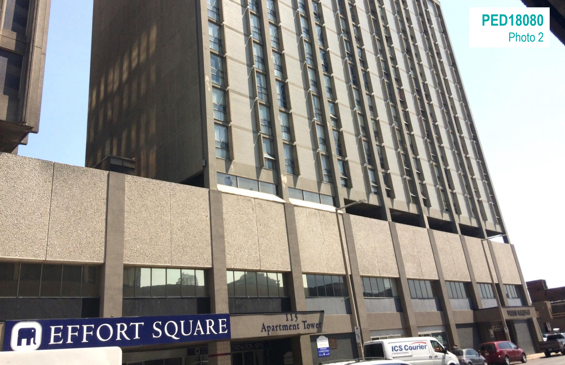
Existing building on the Subject Property as seen from Main Street East looking north
