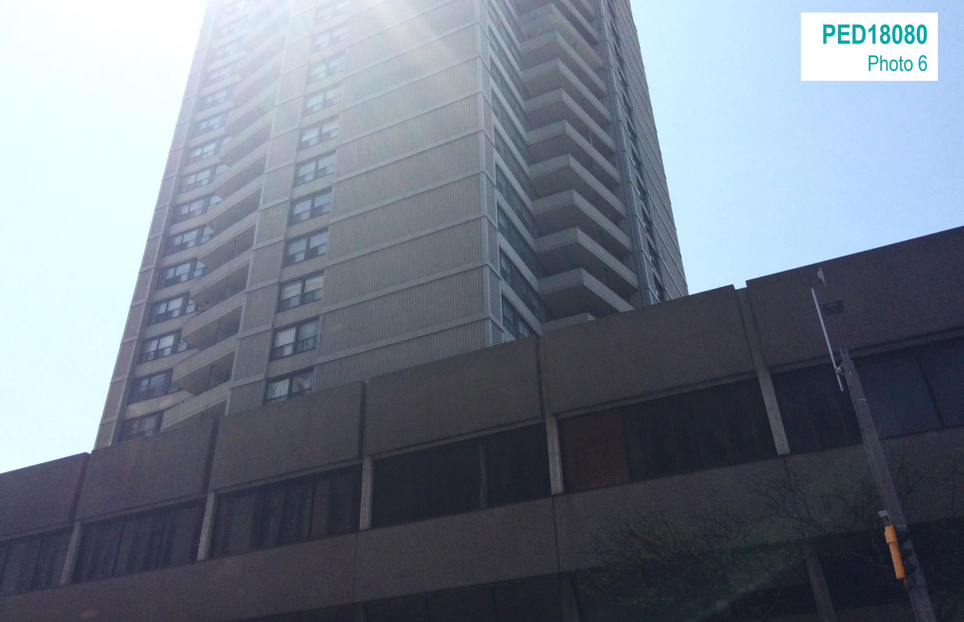
Existing tower of Landmark Place located to the south of the Subject Property, as seen from Main Street East looking south
